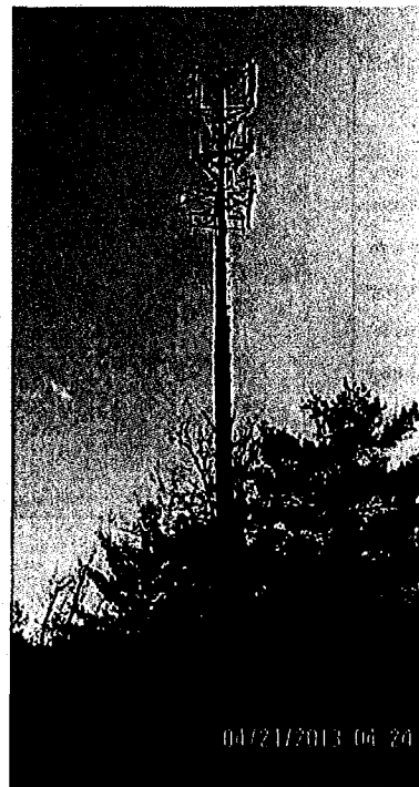
PHOTO OF EXISTING TOWER ELEVATION
