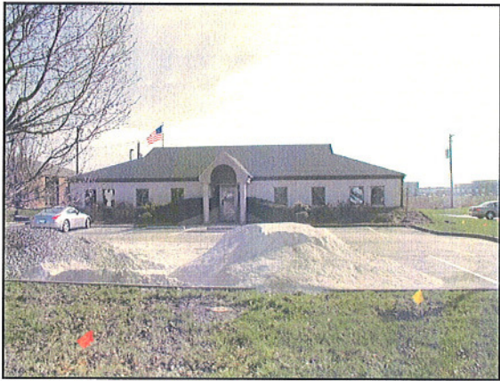
Existing building on site
