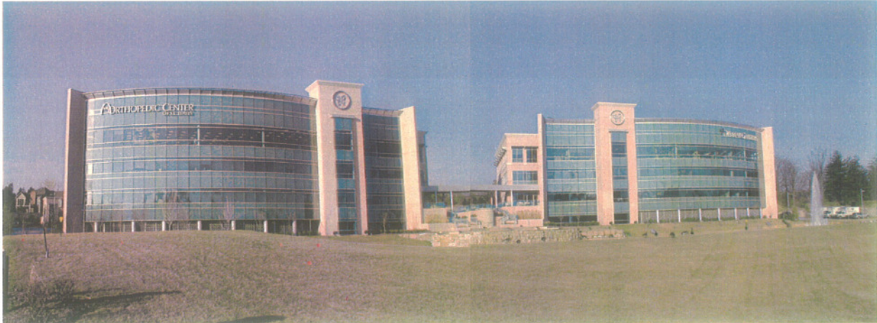
Existing buildings on the site.
