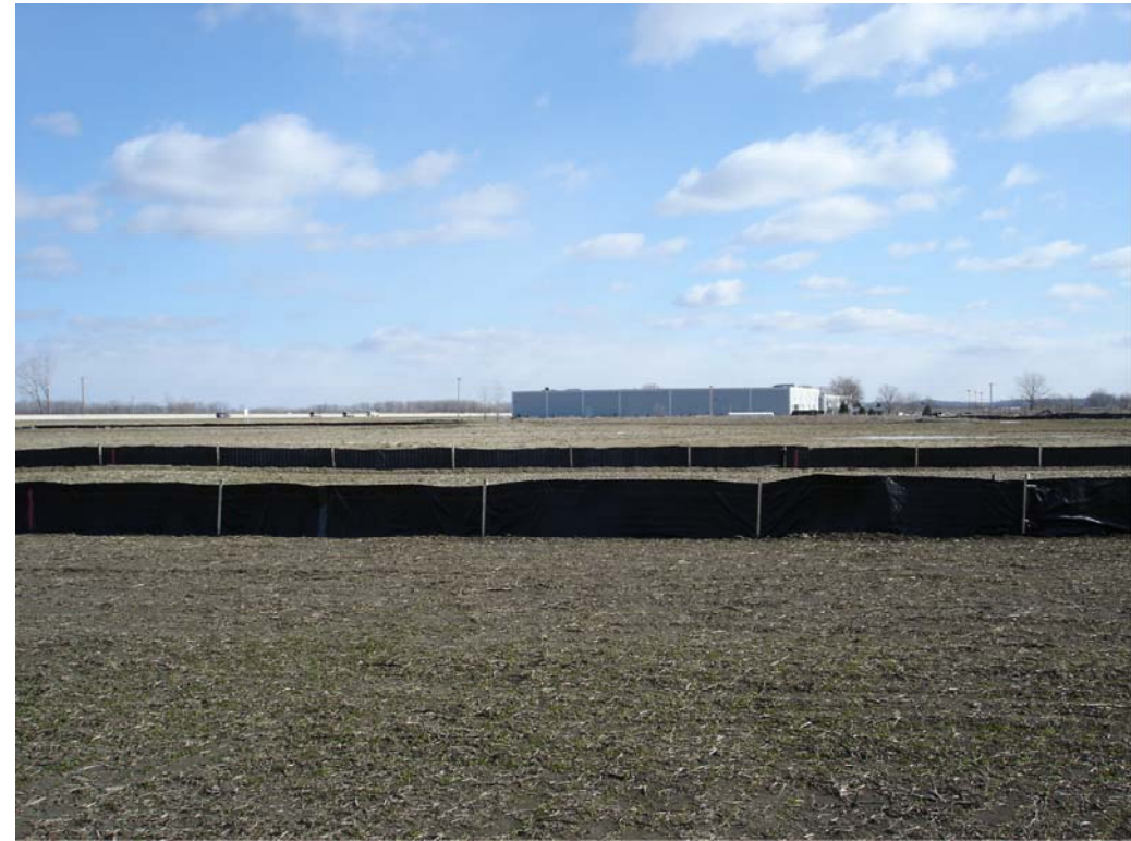
View Looking East
