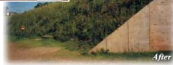
Roadway lane expansion project with reinforced soil slope up to 30 feet tall, spray seeded with native material.
