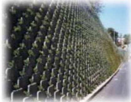
Retail strip center; reinforced wall heights up to 32 feet.
