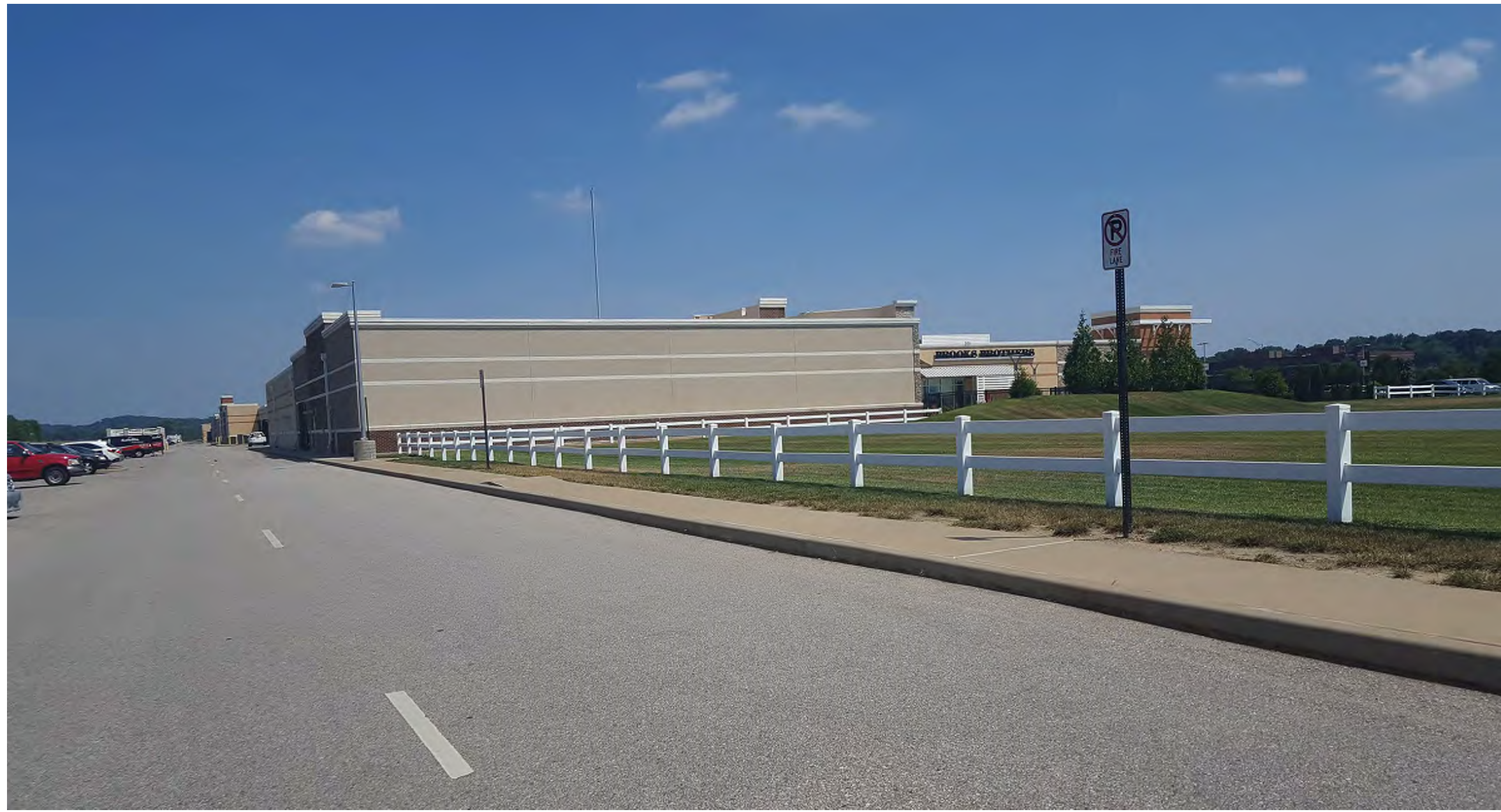
LOOKING SOUTHEAST FROM BACK DRIVE @ NEW BUILDING "A & C"
