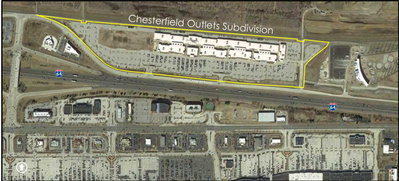
Figure 1: Aerial Site Photo
