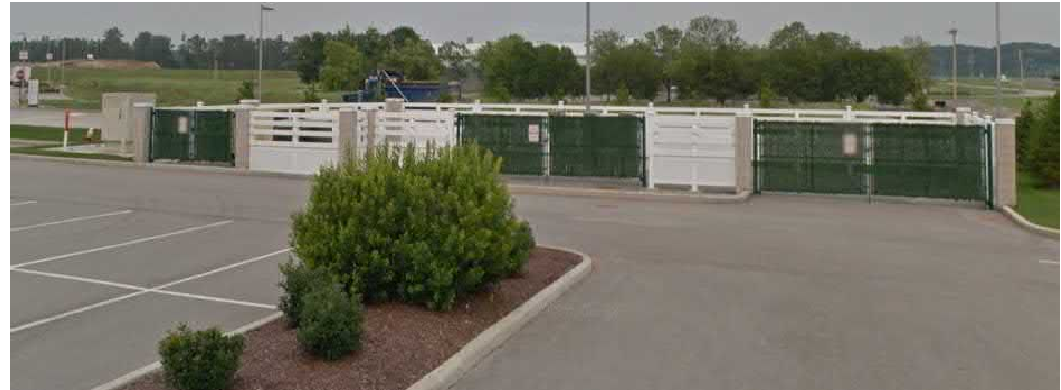
EXISTING SCREENING SYSTEM FOR SANITARY PUMP STATION
