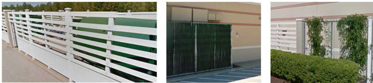
Figure 8: Existing Trash, Electrical Switchgear, and Utility Screening
