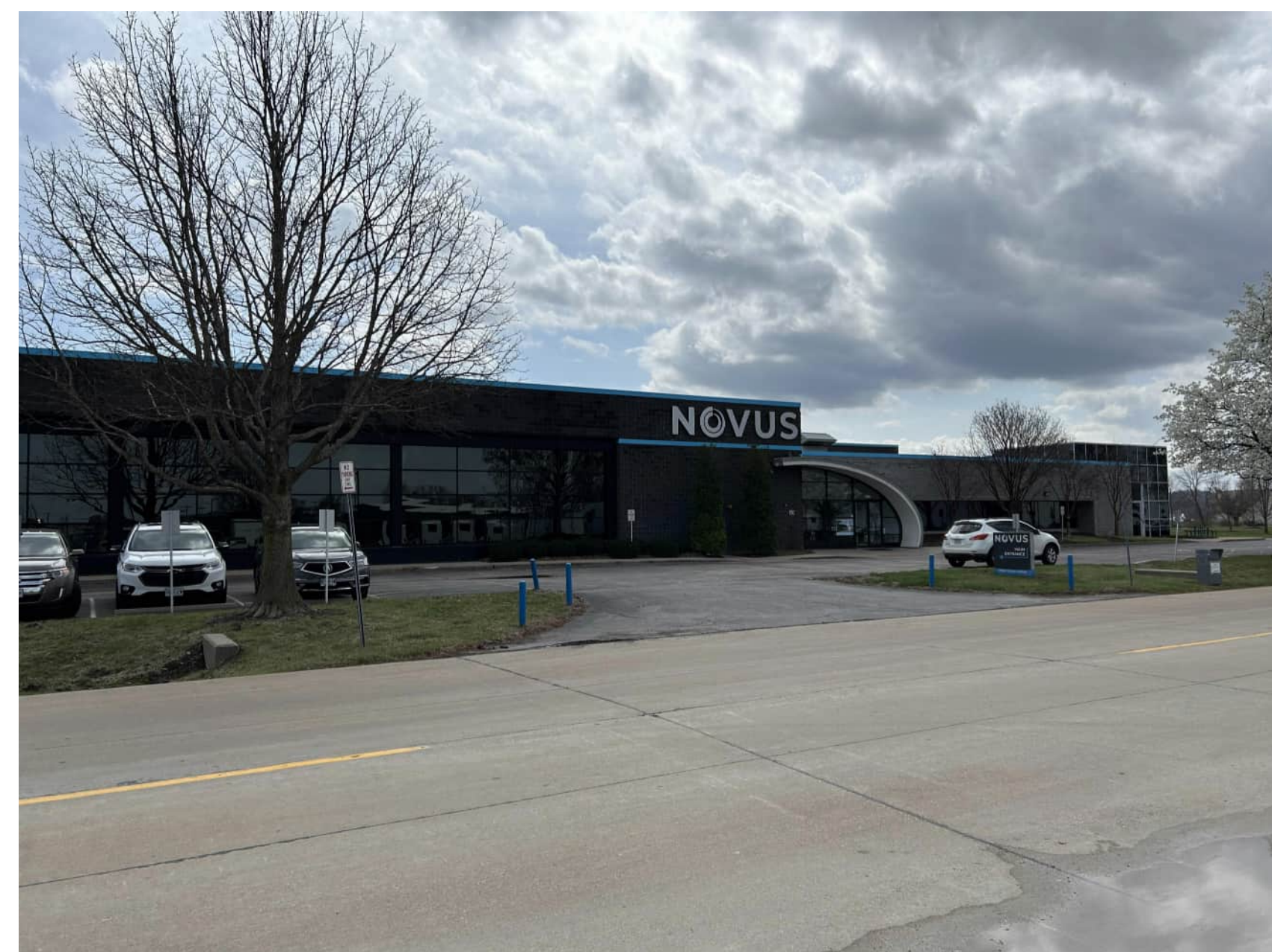
NORTH ELEVATION OF BUILDING
