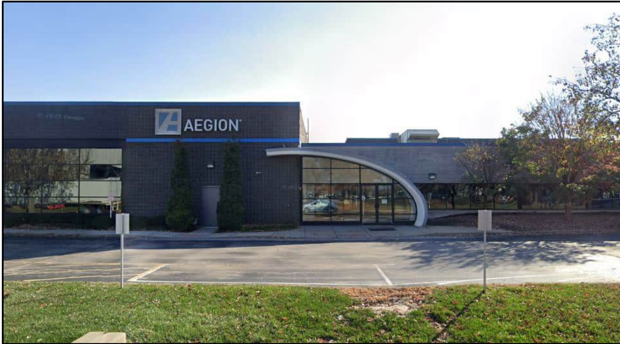
Figure 2: Existing main entrance
