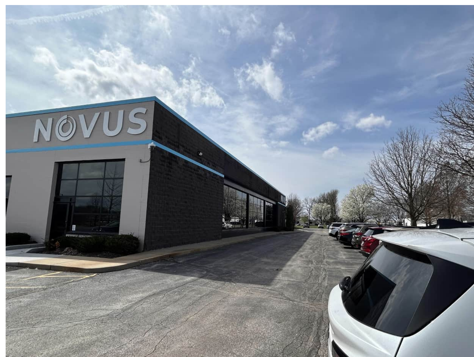
NORTHEAST ELEVATION OF BUILDING
