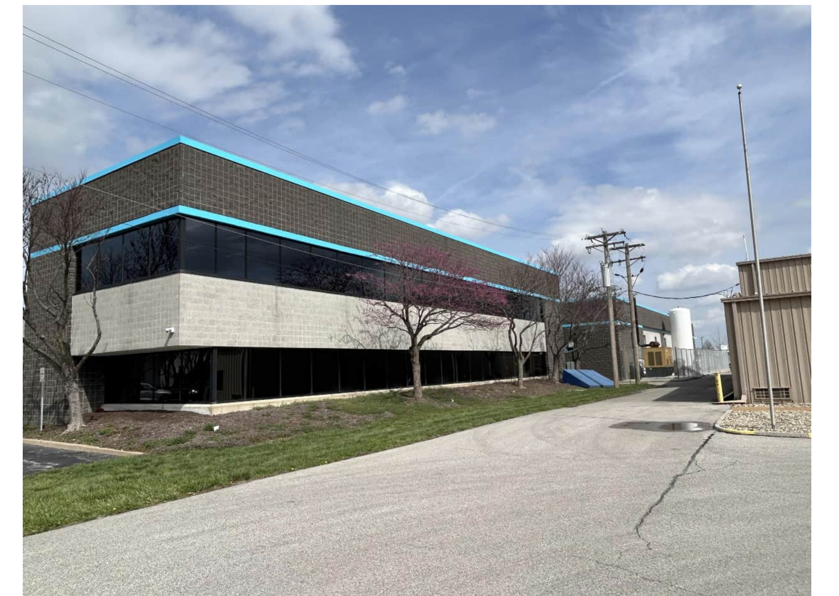
SOUTH ELEVATION OF BUILDING
