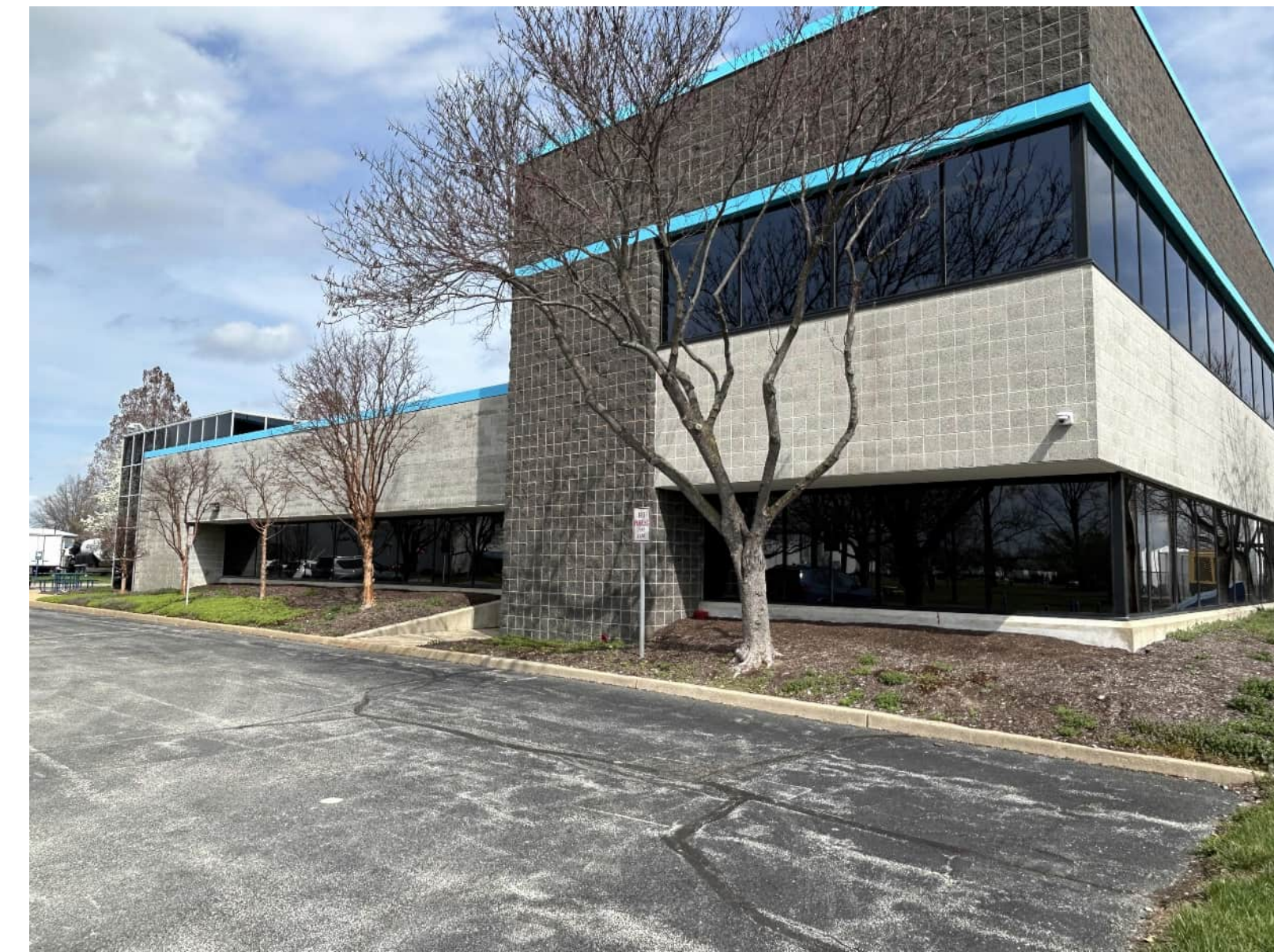
WEST ELEVATION OF BUILDING
