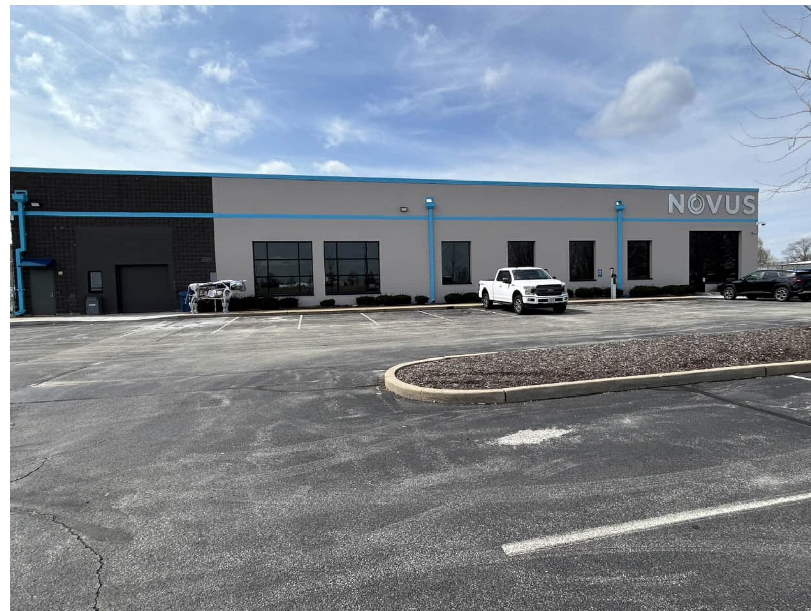
EAST ELEVATION OF BUILDING
