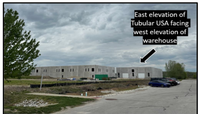
Figure 7: Tubular USA warehouse immediately to the west
