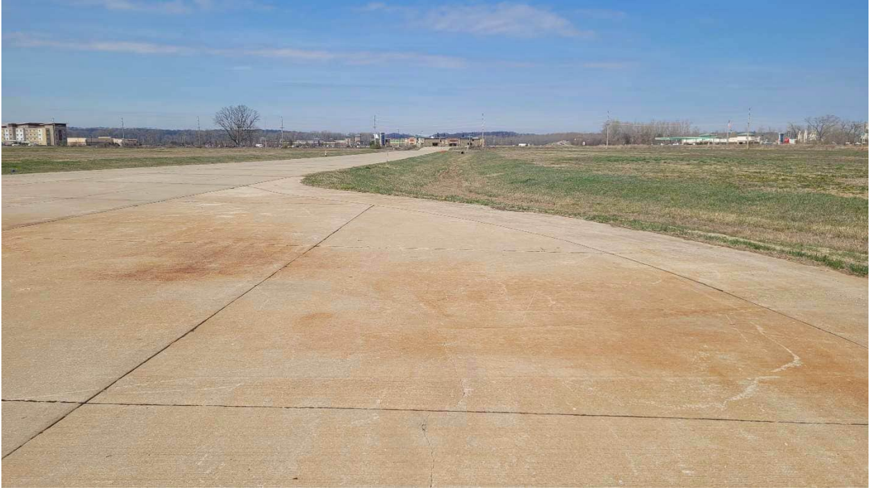
Figure 1 - View from existing Airpark East Cul De Sac, Looking North
