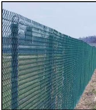
Figure 6: Existing chain-link fence
