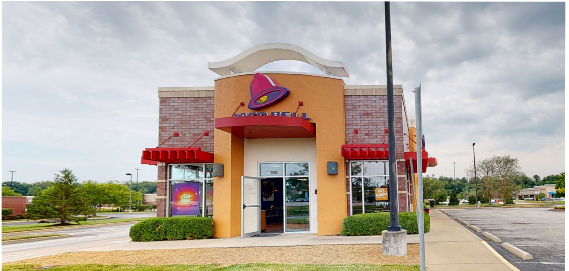
1. BUILDING FRONT – EXISTING
