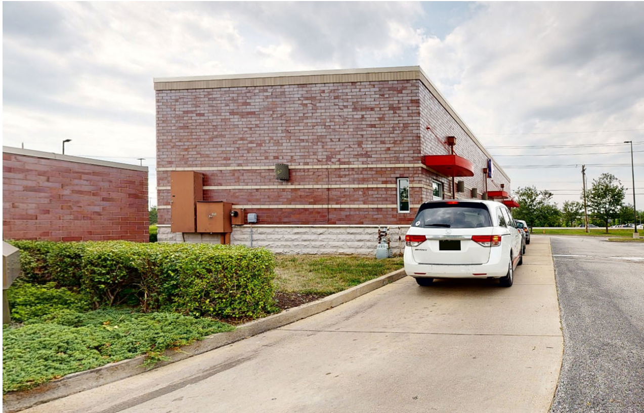
4. BUILDING REAR – EXISTING
