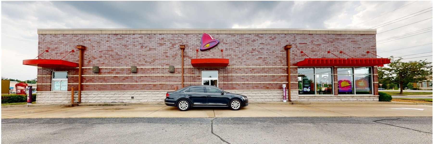
3. BUILDING LEFT – EXISTING
