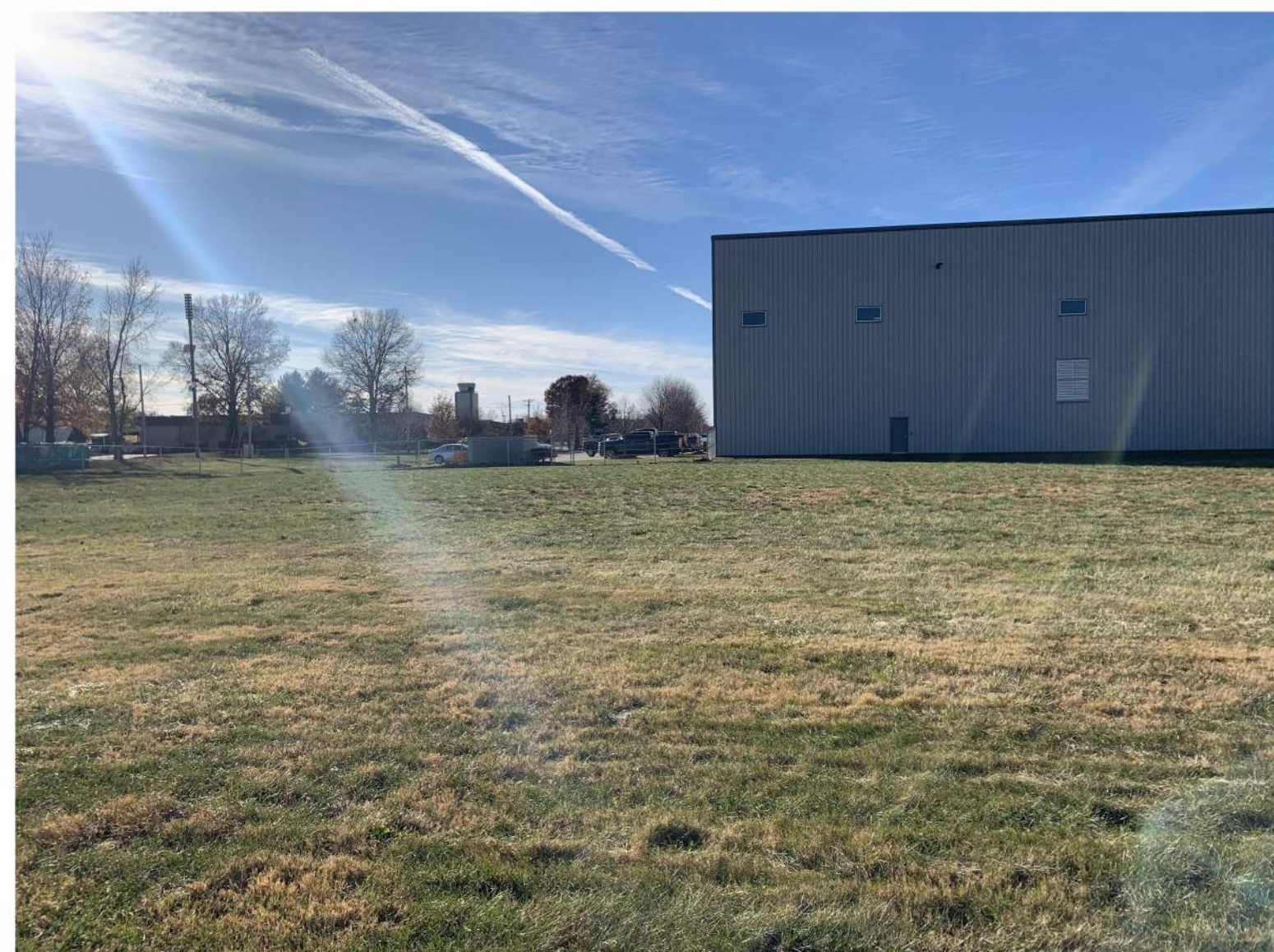
VIEW LOOKING SOUTHWEST
