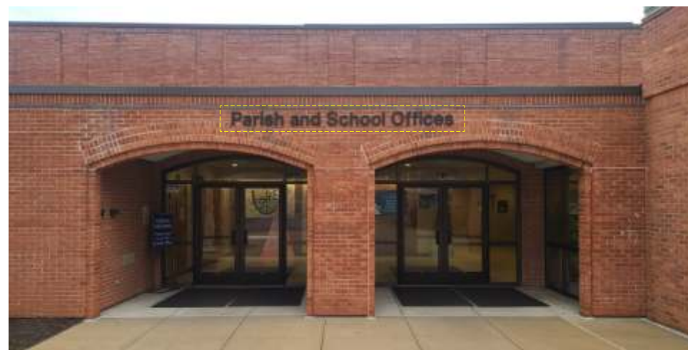
LETTERS ON WALL - 8.5" H x 142" W (8.4SF) EXISTING WALL SIGNS ON PROPERTY
