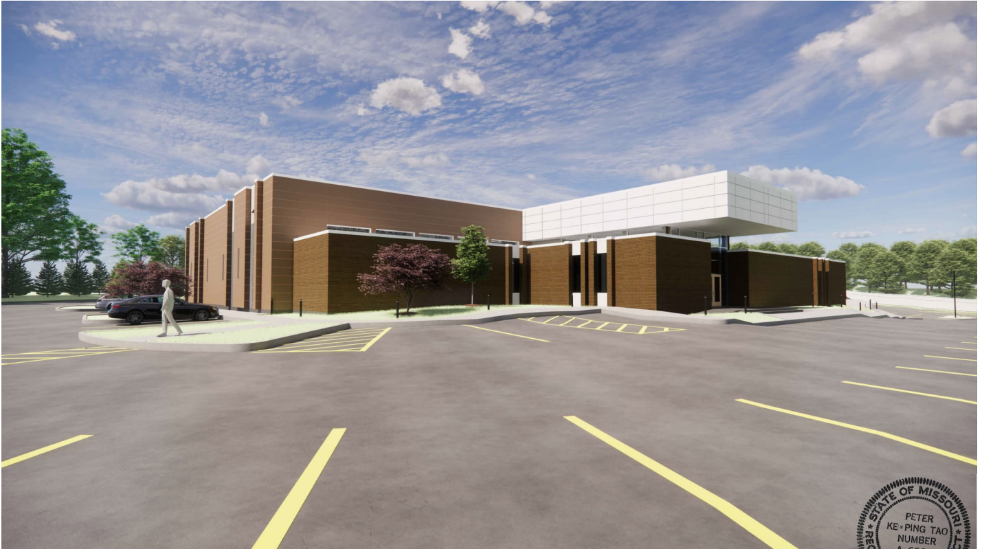
EXISTING MAIN ENTRY AND FRONT OF ADDITION
