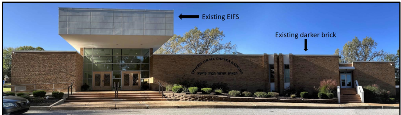
Figure 4: Existing conditions of north elevation
