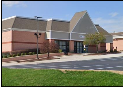
Figure 2: Existing front façade
