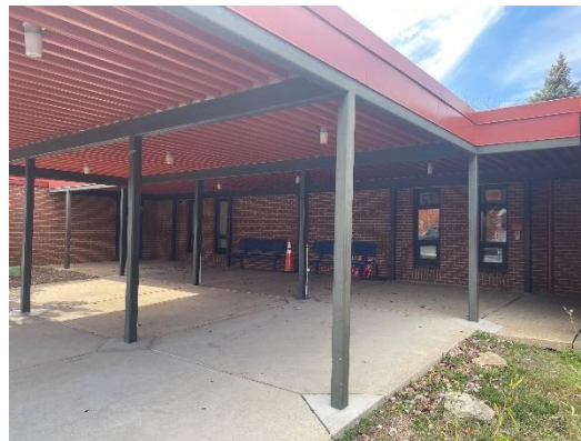
Figure 3. Existing Front Entrance
