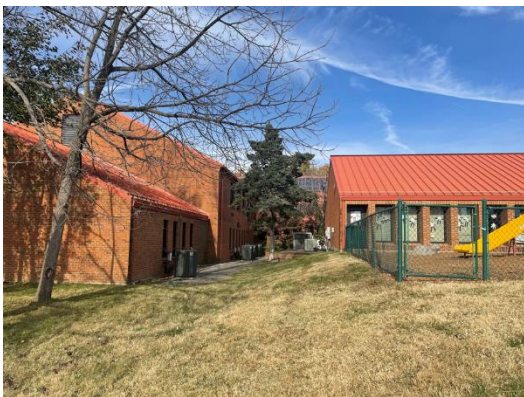
Figure 2. Area between new additions for ADA ramp to Storm Shelter below grade.
