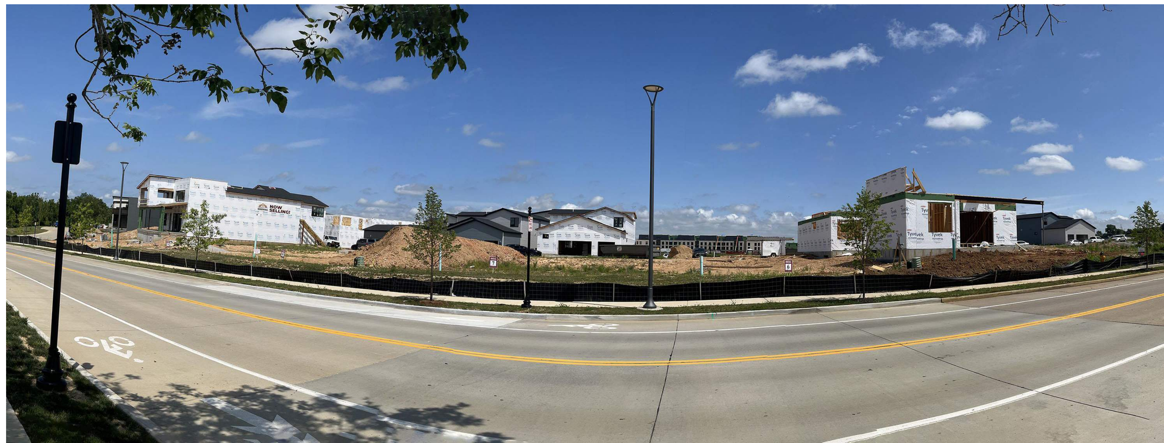
SITE PHOTO LOOKING NORTH
