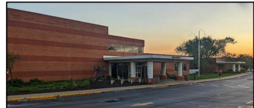
Figure 4: Existing North Façade (Left View)
