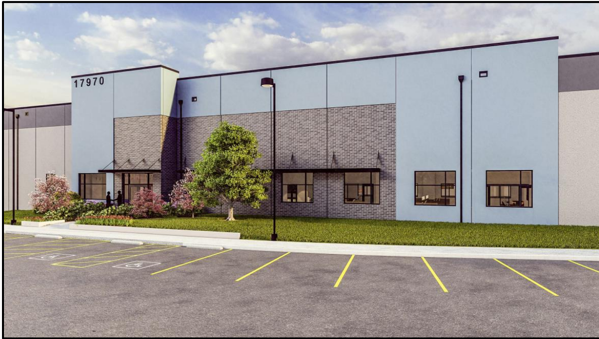
Figure 7: View of Main Entry
