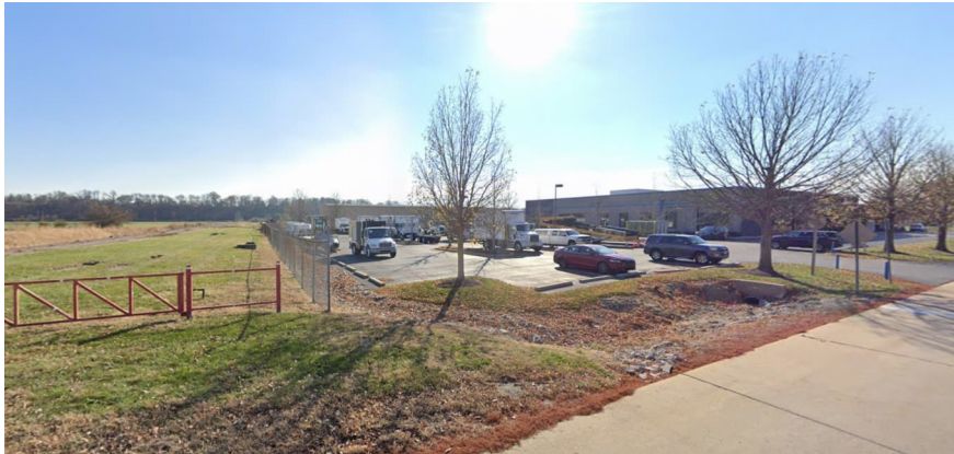
17988 EDISON AVE. - AGEION HEADQUARTERS
