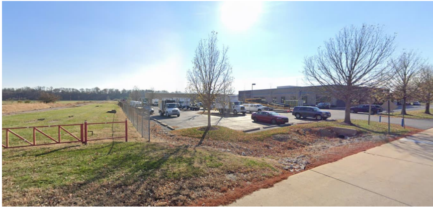
17988 EDISON AVE. - AGEION HEADQUARTERS
