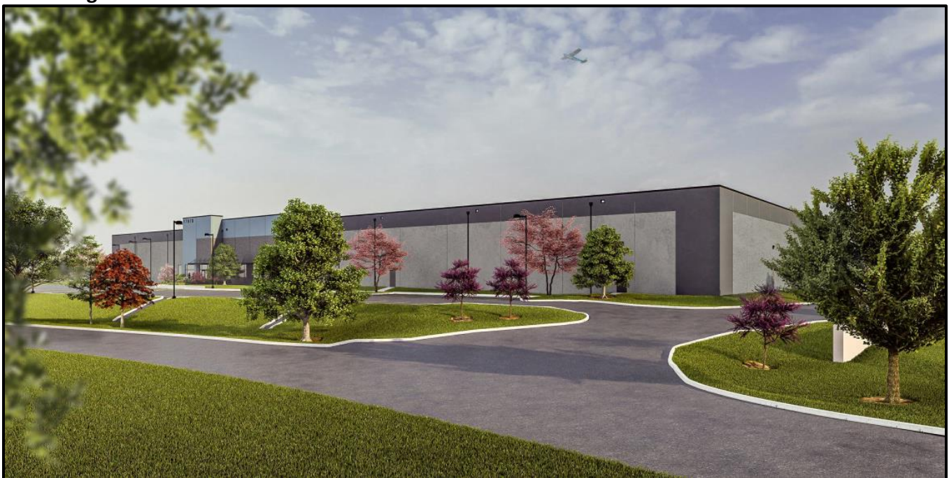
Figure 6: View from Edison Avenue
