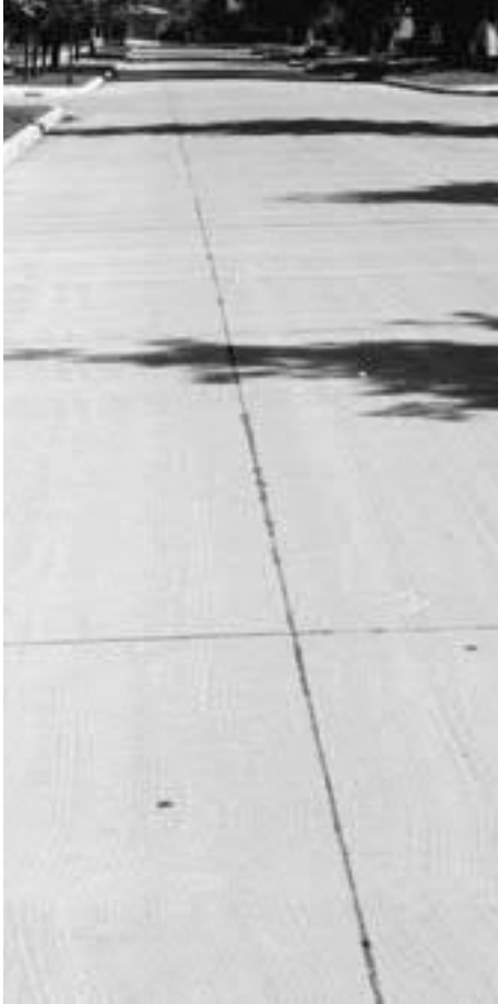
◀ New, well-sealed longitudinal joint.
