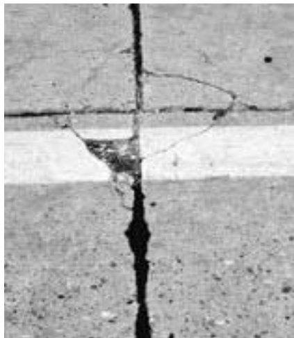
First signs of corner cracking.
