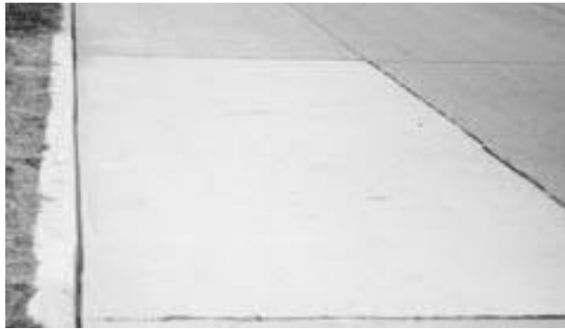
◀ Extensive pop-outs. Pavement is unsightly but still provides good level of service.
