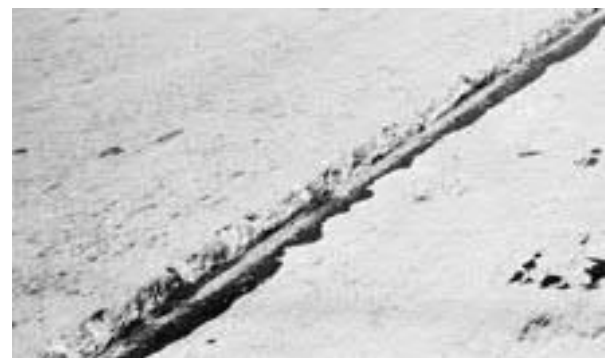
▲ Faulted longitudinal joint.
