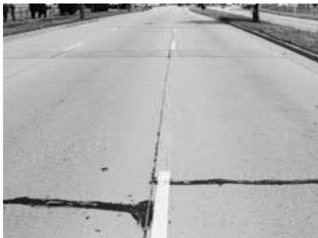
◀ Transverse crack. Tight, sound pavement.
