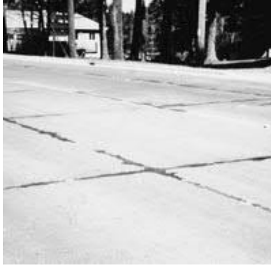
▼ Corner crack with spalling.
