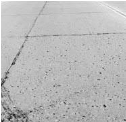
◀ Extensive pop-outs. Pavement is unsightly but still provides good level of service.
