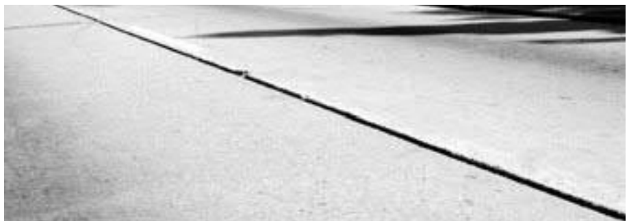
▲ Faulted longitudinal joint.
