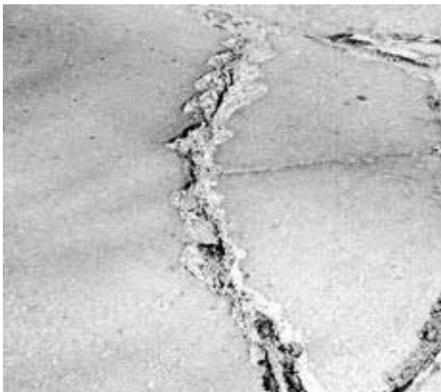
▶ Spalling over shallow reinforcing.
