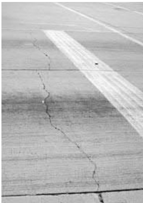
◀ Transverse crack. Tight, sound pavement.
