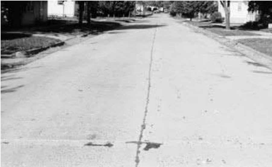
◀ Extensive pop-outs. Pavement is unsightly but still provides good level of service.
