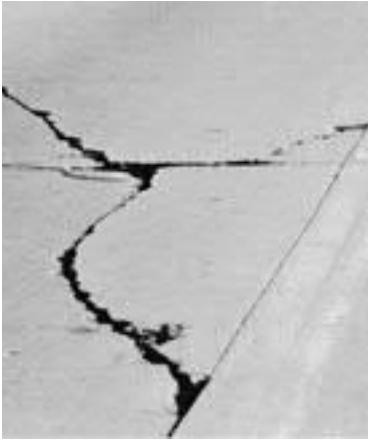
▼ Corner crack with spalling.
