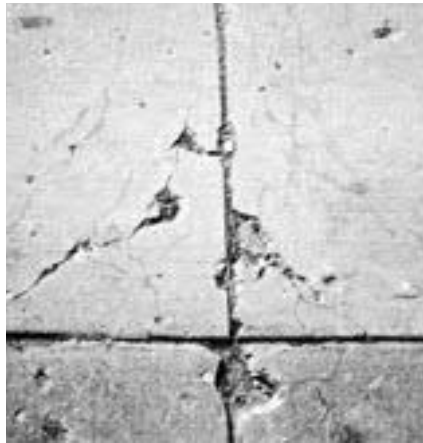
Corner cracking with broken concrete pieces.
