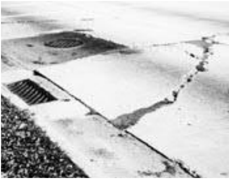
▲ Remove and replace pavement around manhole and inlet.
