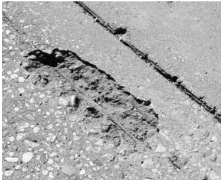
▶ Spalling over shallow reinforcing.
