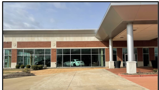
Figure 5: Portion of the existing east elevation
