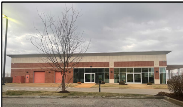
Figure 4: Existing south elevation
