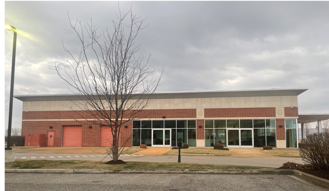
SOUTH ELEVATION - OVERALL
