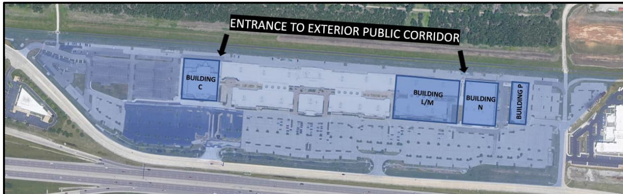
Figure 2: These buildings are generally set up for a single occupant and are visible to the public realm and/or Interstate 64.
