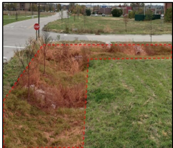
Figure 6: Drainage area along northeast corner of site
