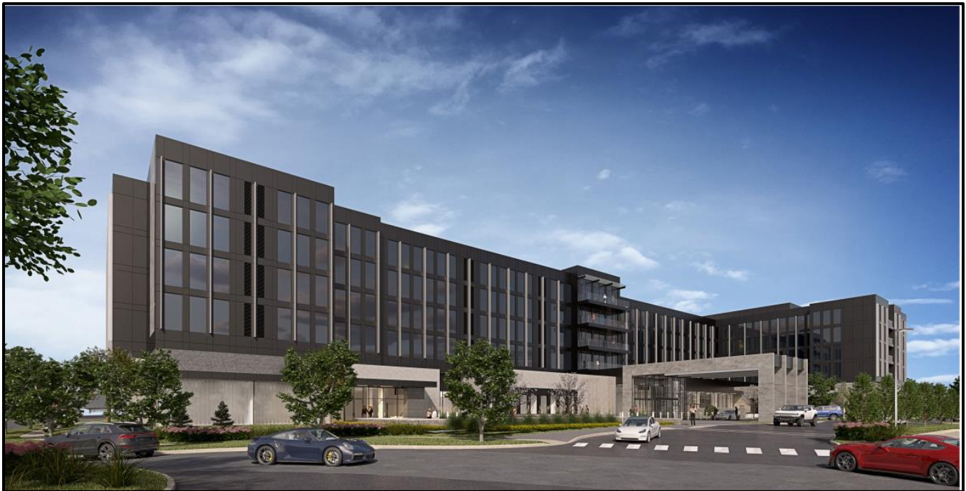
Figure 8: View from internal drive
