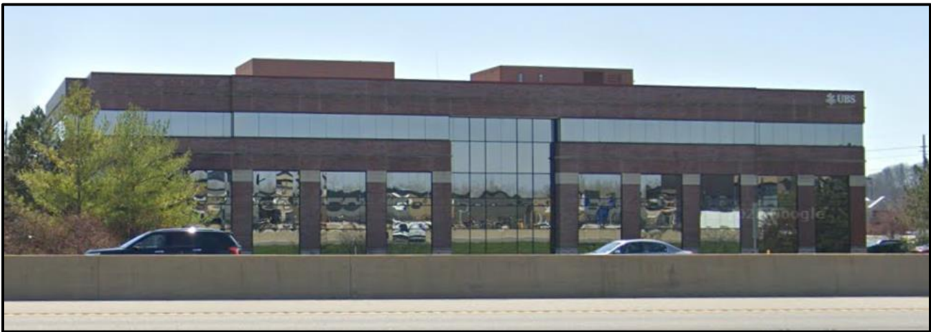
Figure 3: North Elevation facing I-64
