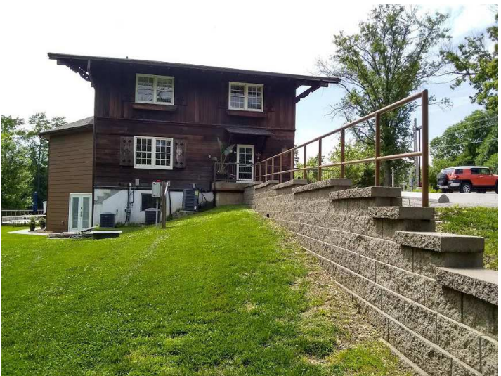
EXISTING RETAINING WALLS
