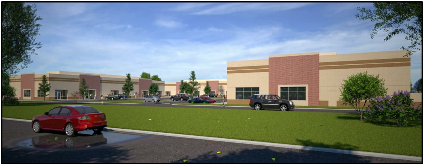
Figure 8: Service Center Buildings
