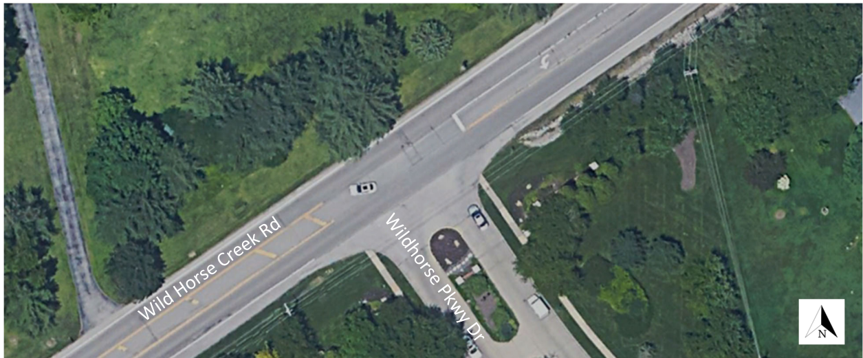
Figure 2: Aerial of Wild Horse Creek Road at Wildhorse Parkway Drive Intersection
