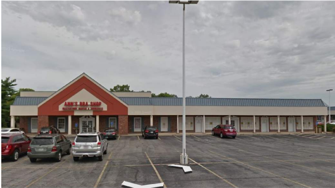
BUILDING TO NORTH OF PROPERTY
