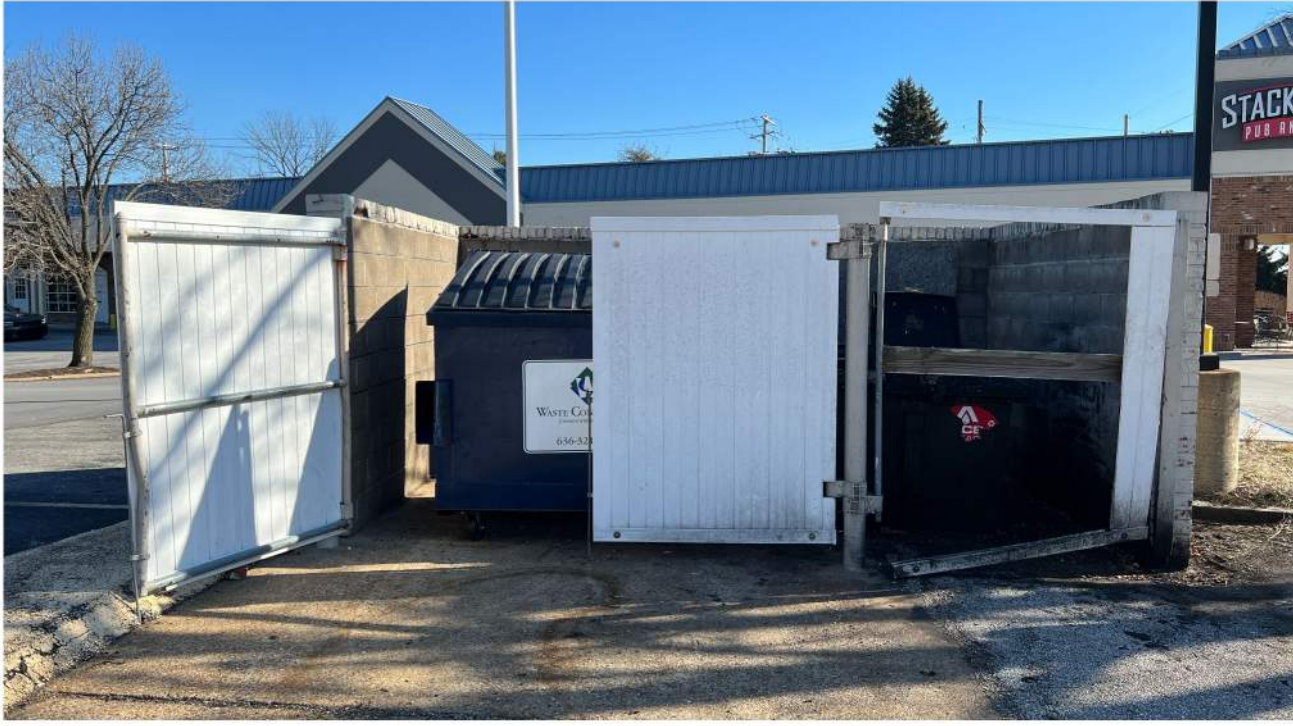
PHOTO OF EXTG. TRASH ENCLOSURE
