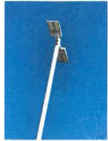
Closeup of existing double head LED light fixture
