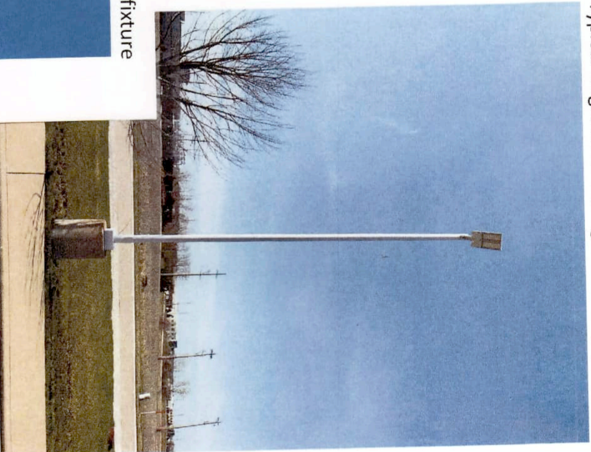
Typical single head LED light fixture @ perimeter
