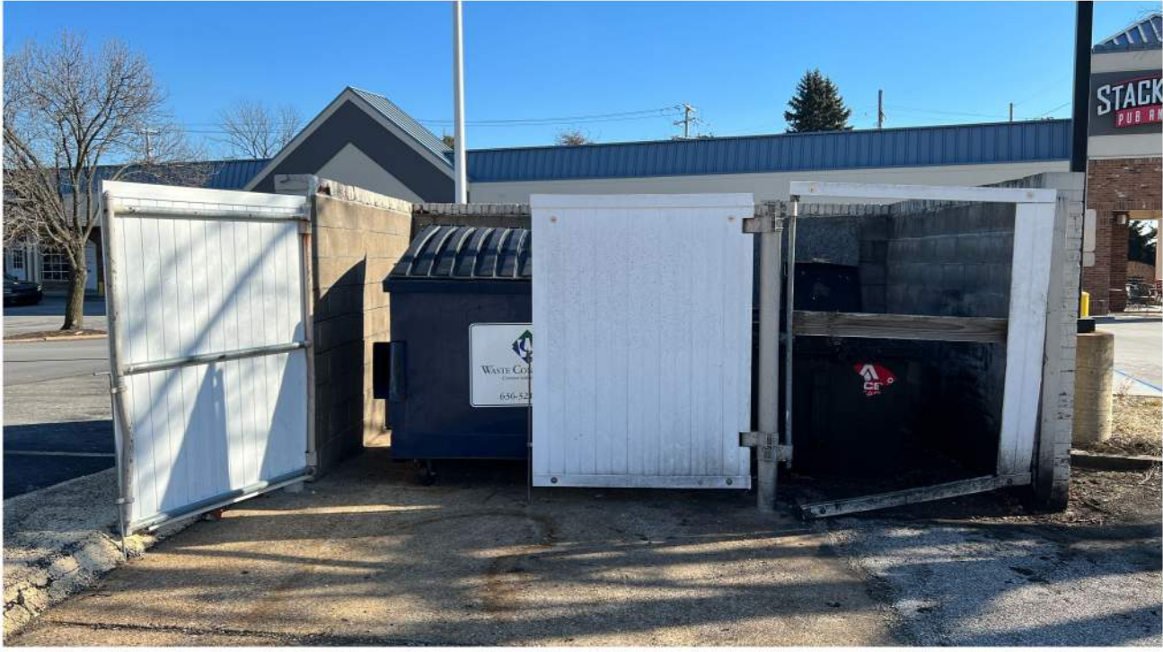
PHOTO OF EXTG. TRASH ENCLOSURE
