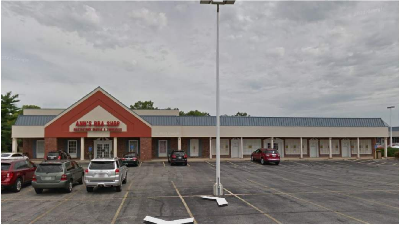
BUILDING TO NORTH OF PROPERTY
