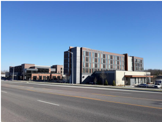
AC HOTEL CHESTERFIELD - NORTH OF SITE
