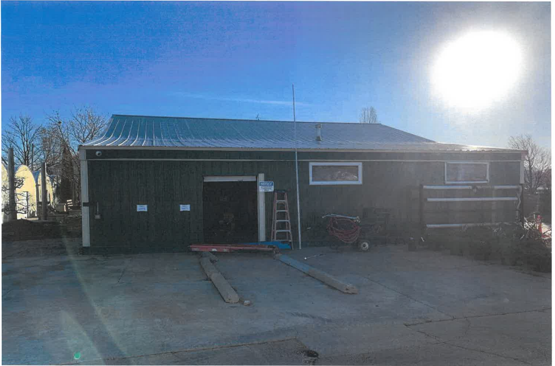
Building: Shed, side 3 Height: 10'
