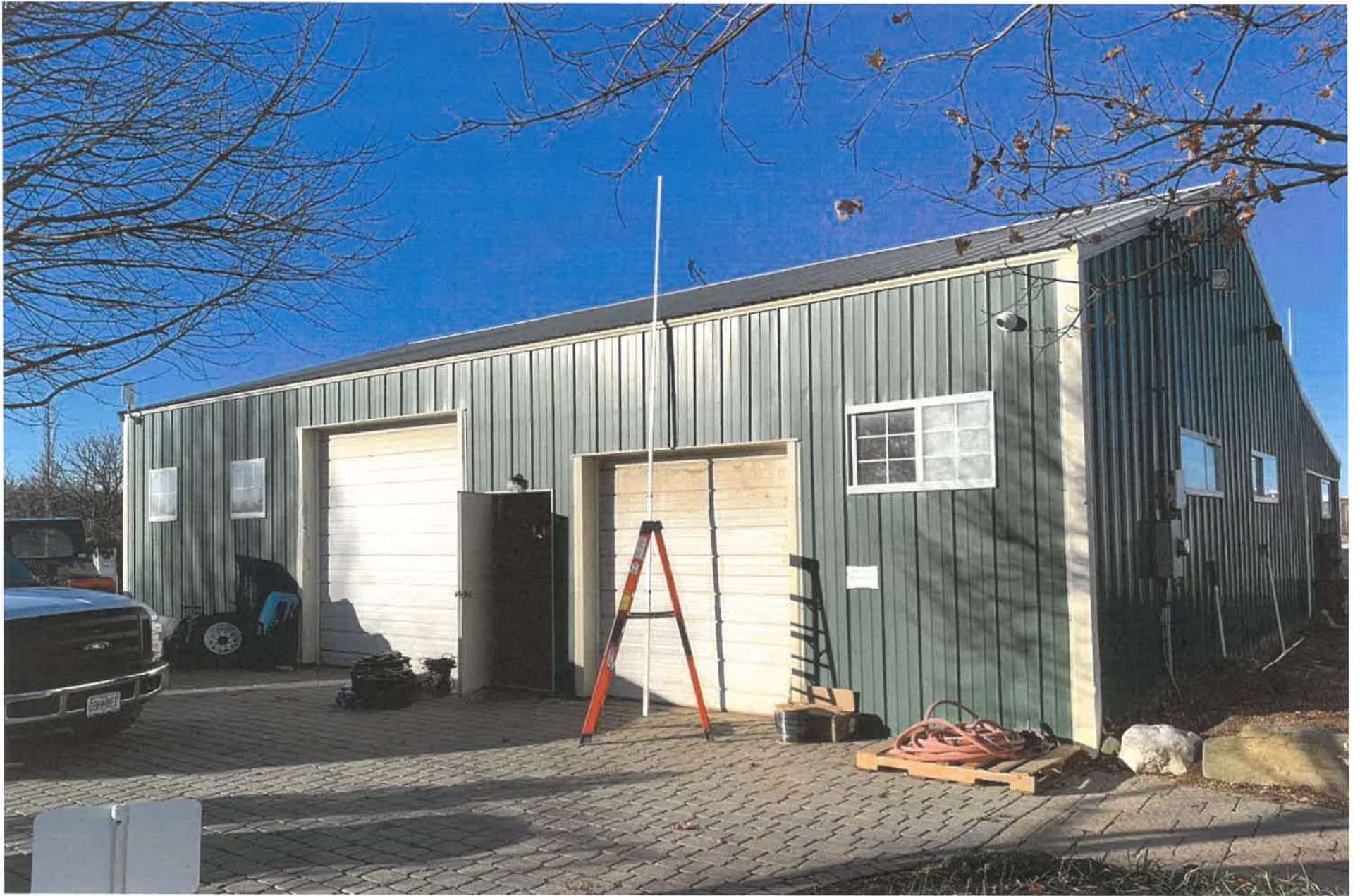
Building: Shed, Side 1 Height: 12'
