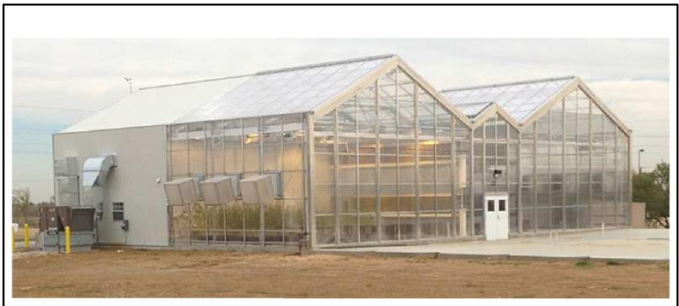
Figure 10: Greenhouse Addition (Existing Utility Building)
