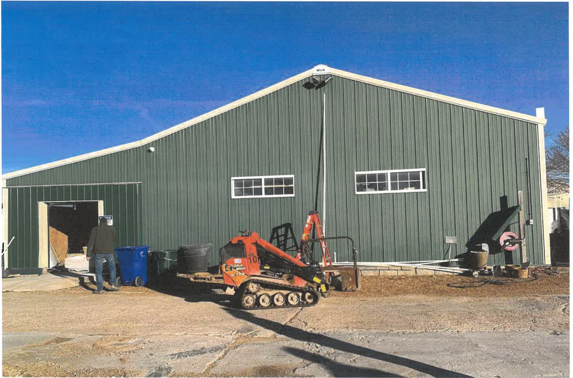
Building: Shed, side 2
