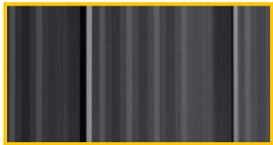
EXISTING STANDING SEAM METAL ROOF
