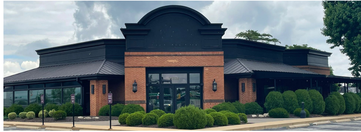
EXISTING EXTERIOR -SOUTH
