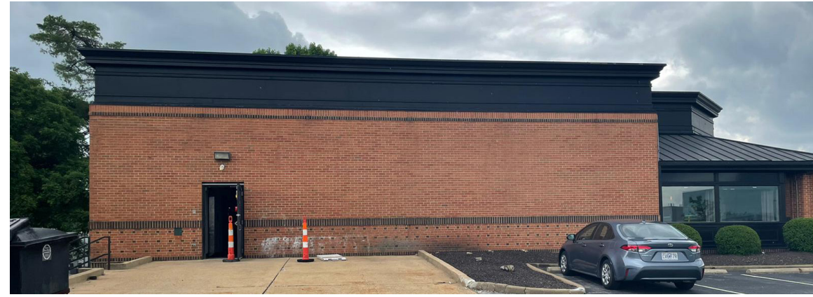
EXISTING EXTERIOR -NORTH WEST
