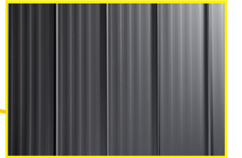
Standing Seam Roof
