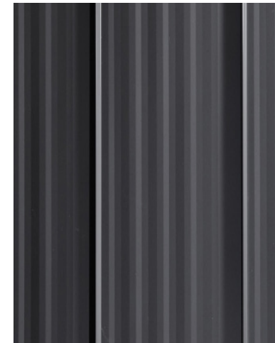
Existing Standing Seam Metal Roof
