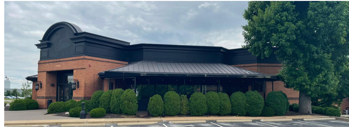
EXISTING EXTERIOR -SOUTH EAST
