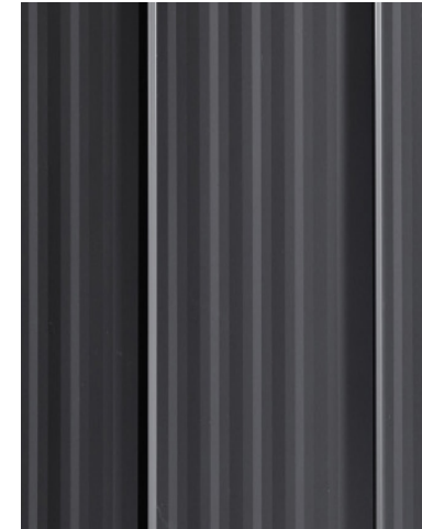
Existing Standing Seam Metal Roof
