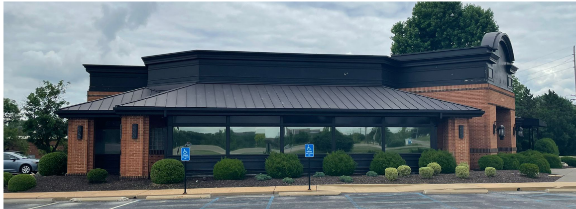
EXISTING EXTERIOR- SOUTH WEST
