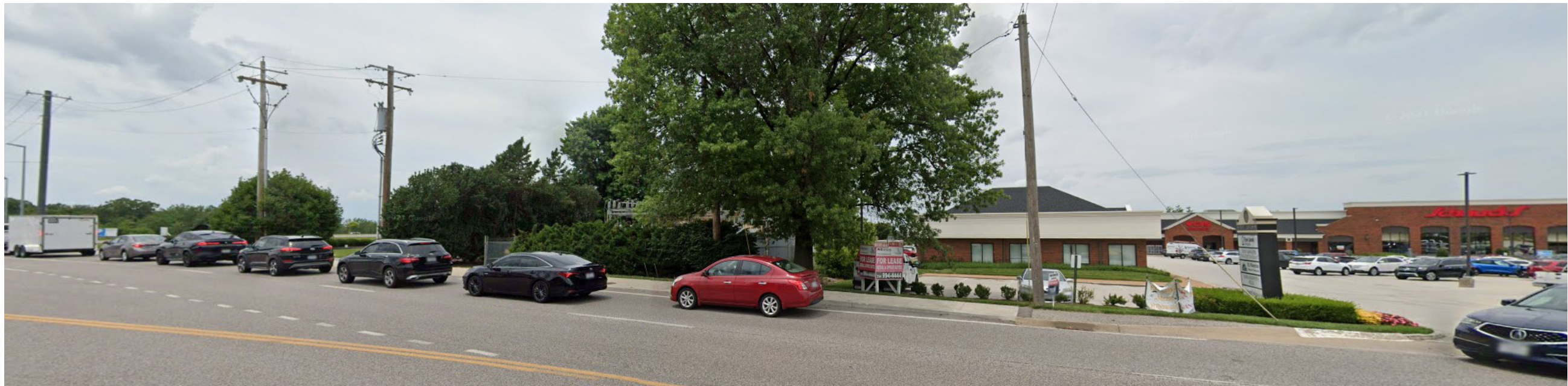
OLIVE BLVD LOOKING NW TOWARD SITE
