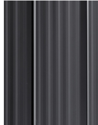
Existing Standing Seam Metal Roof
