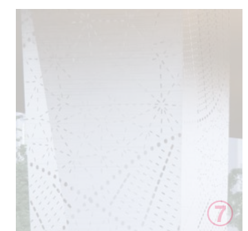
METAL PANEL-CLAD COLUMNS
