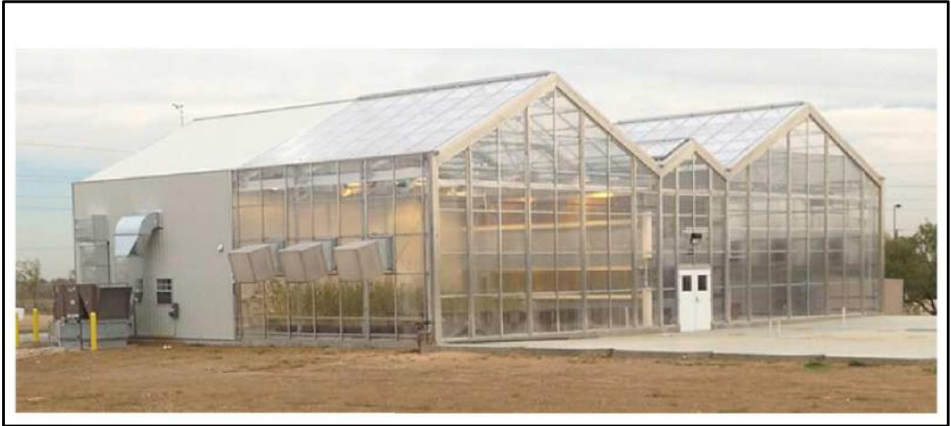
Figure 8: Greenhouse Addition (Existing Utility Building)
