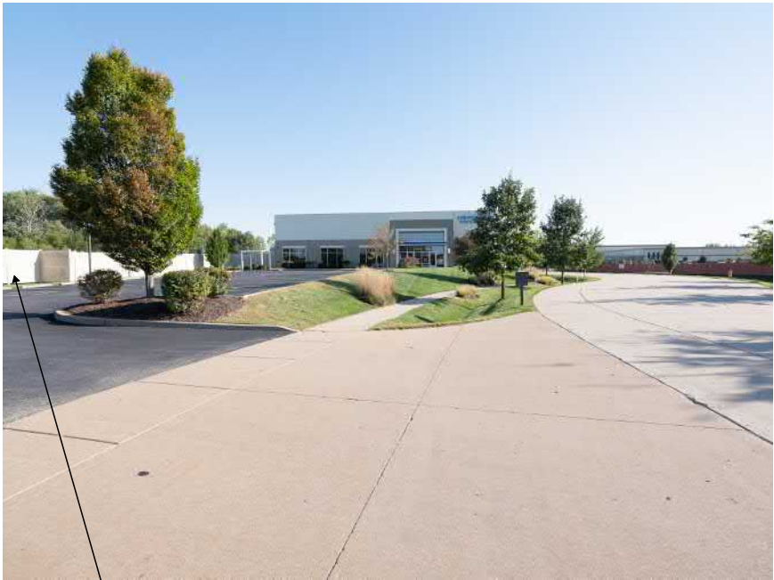
Spirit Valley East Drive (looking south) - Industrial office / workshop / equipment & material storage
