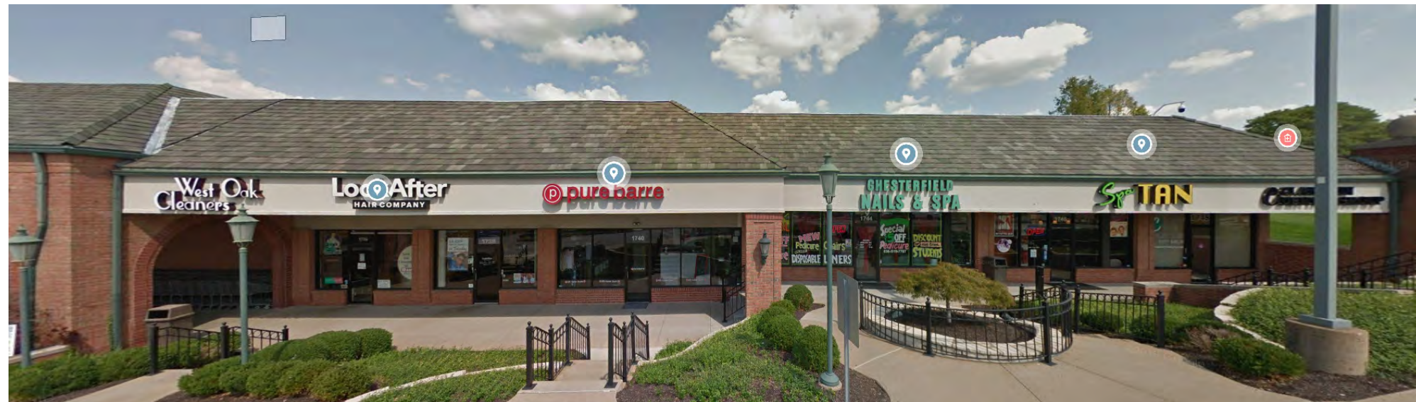
EXISTING ADJACENT PROPERTY PHOTOS
