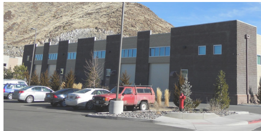
Wall recesses, height variations, material changes and repeating patterns along the entire facade.
