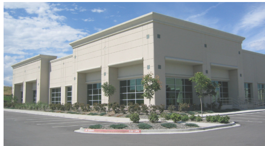
Wall projections/recesses, height variations and repeating patterns along the entire facade.
