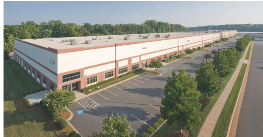
Wall projections and repeating patterns along the entire facade.
