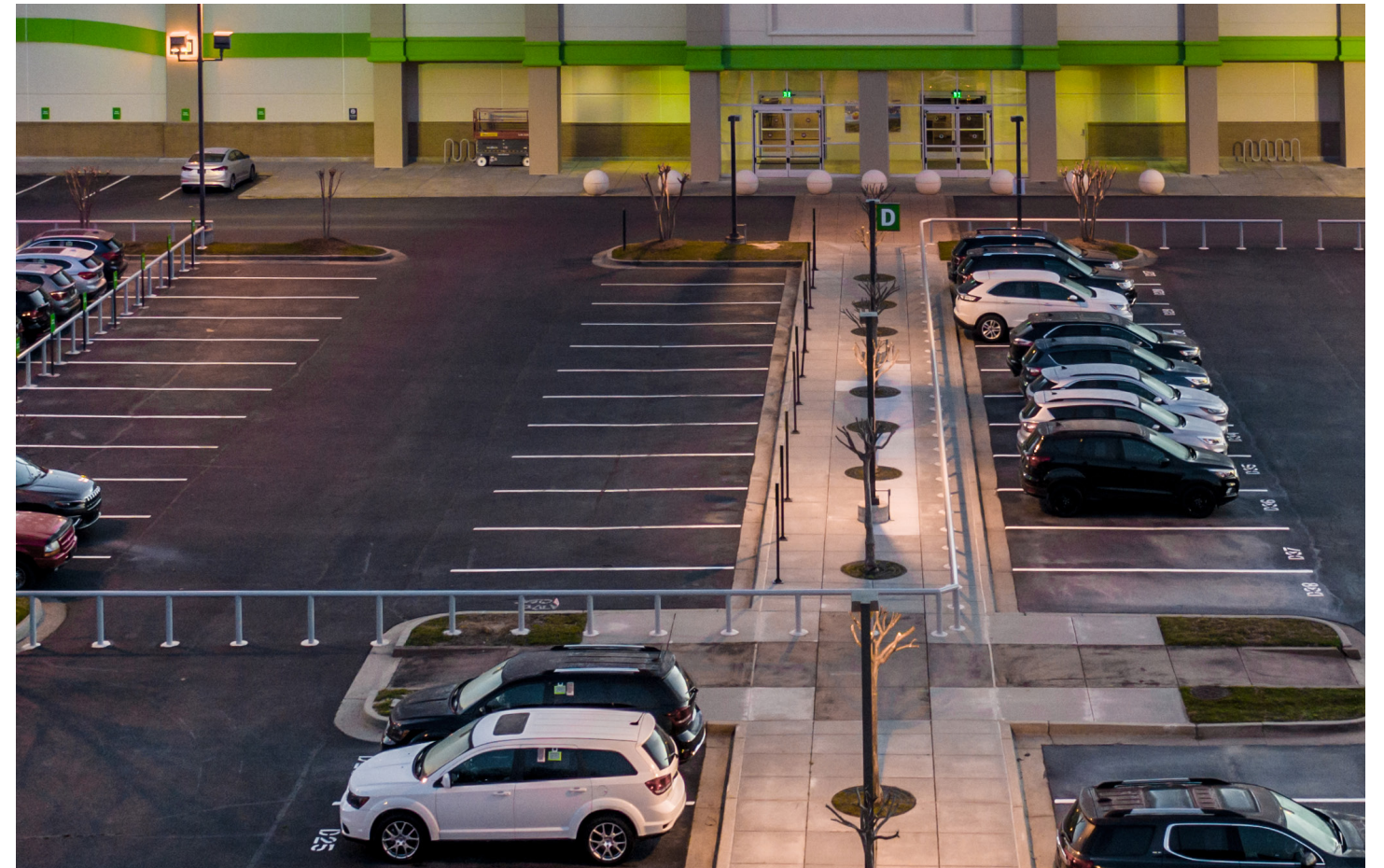
Bollard Rail Implemented at Echo Park Store
