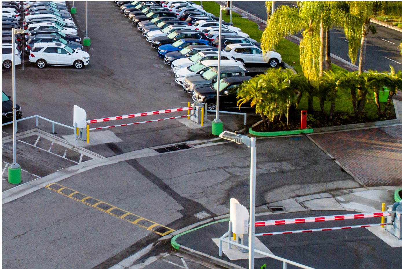
Non-Illuminated Security Gate at Echo Park Store
