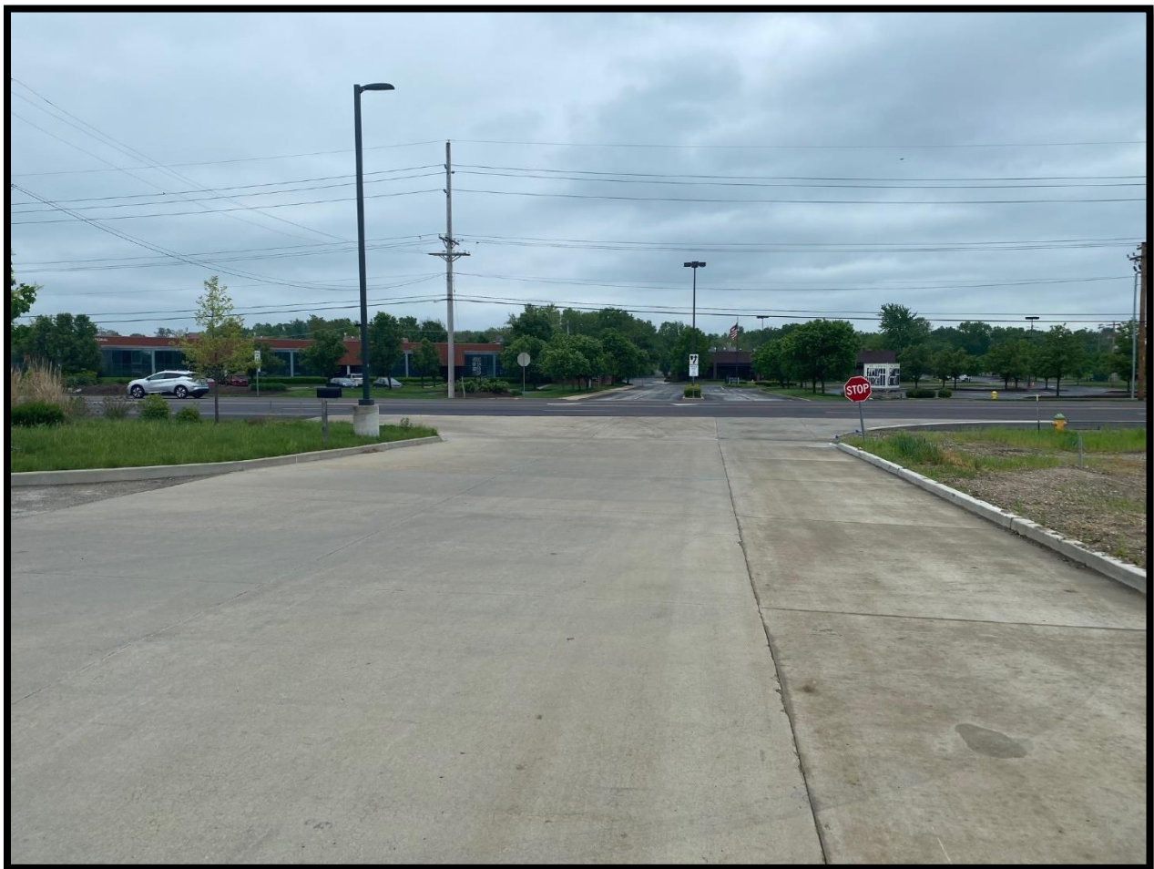
Figure 11. Southbound Approach of Drive Adjacent to AutoZone to Chesterfield Airport Road
