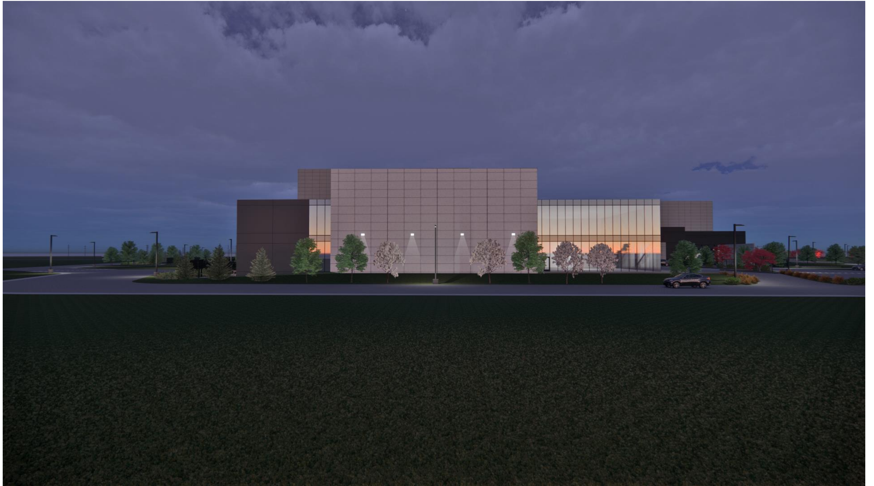
STUDIO 2 FACING INTERSTATE
