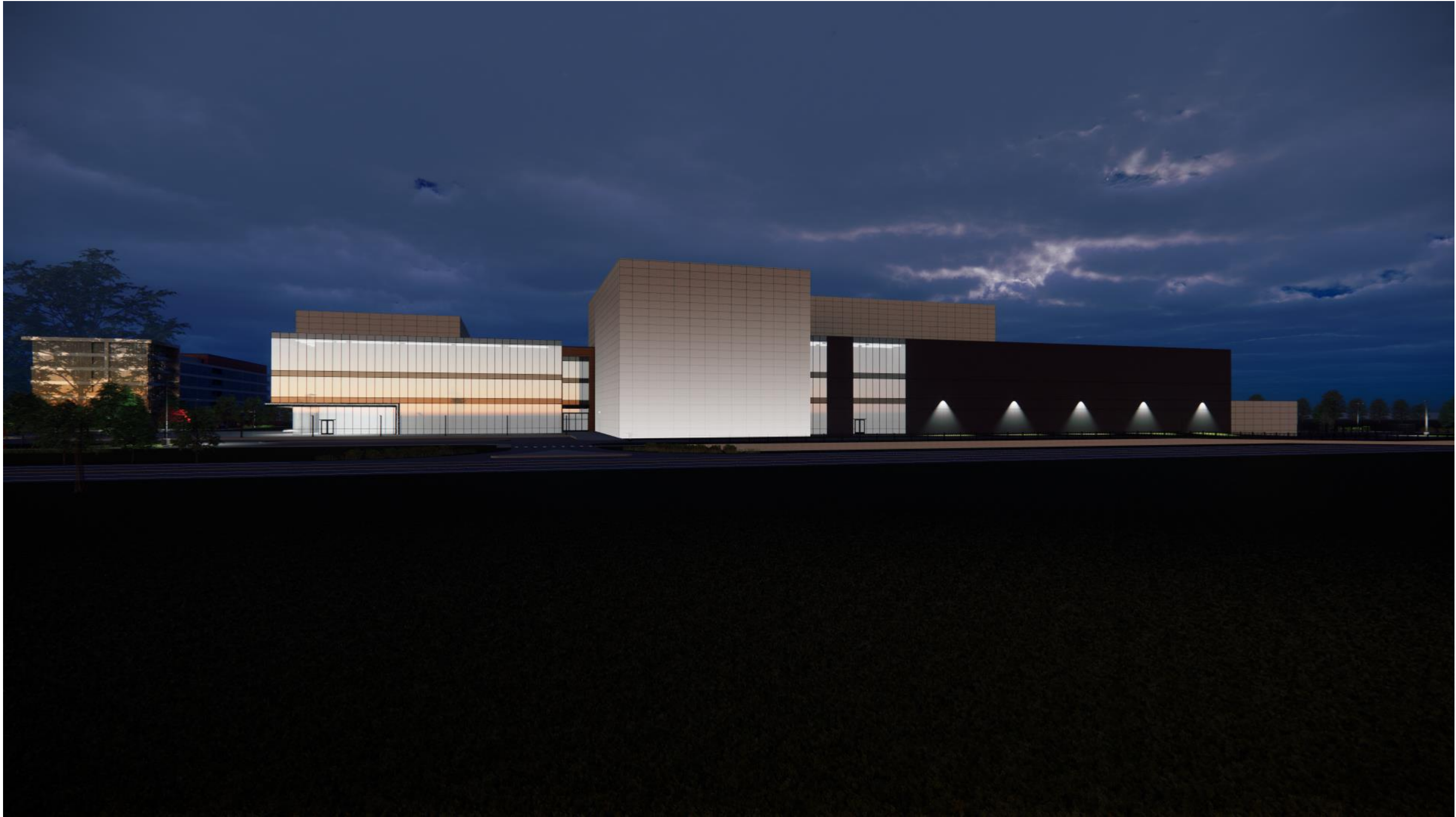
MAIN BUILDING: FRONT FAÇADE FACING CHESTERFIELD AIRPORT ROAD
