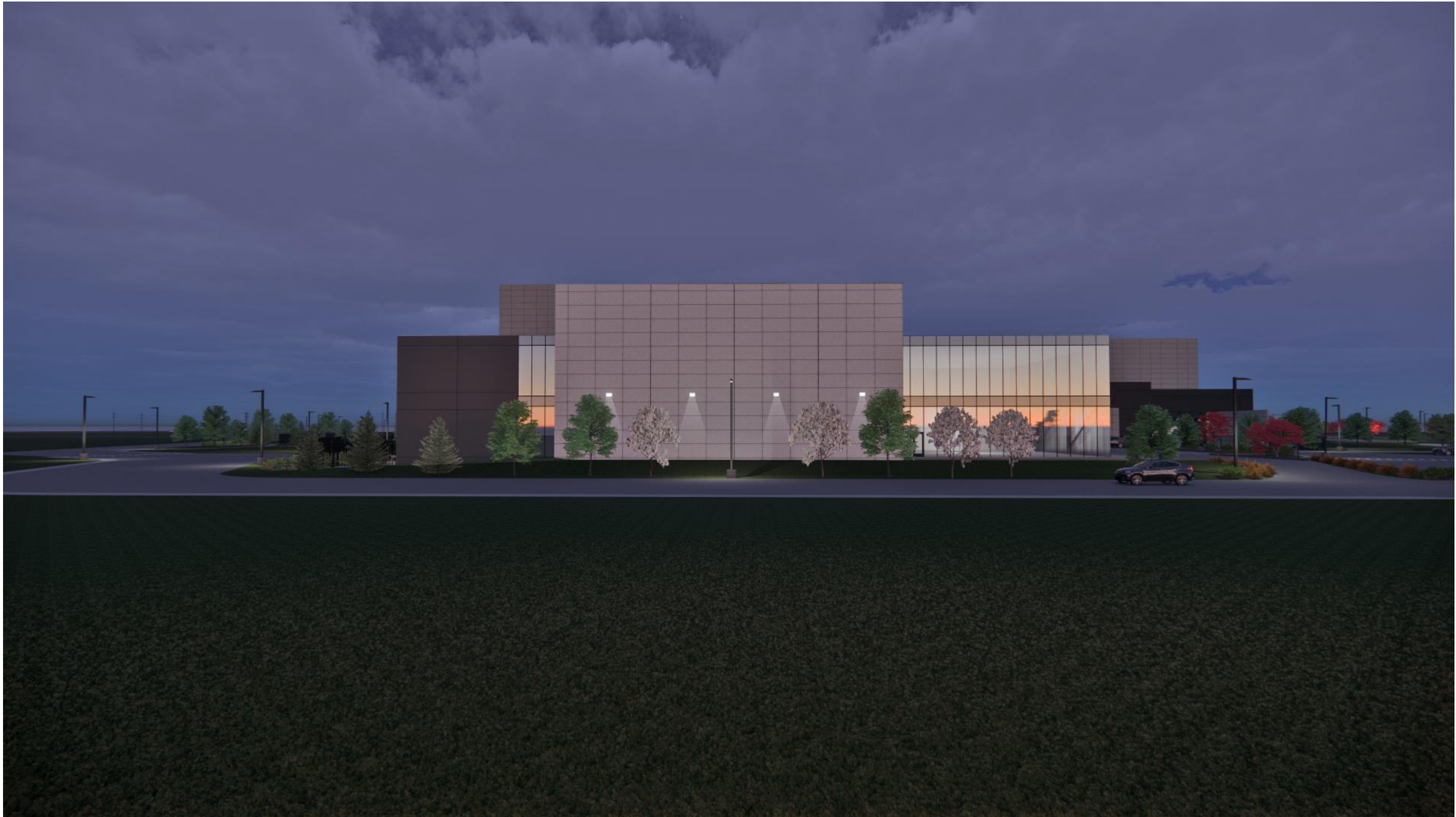
STUDIO 2 FACING INTERSTATE
