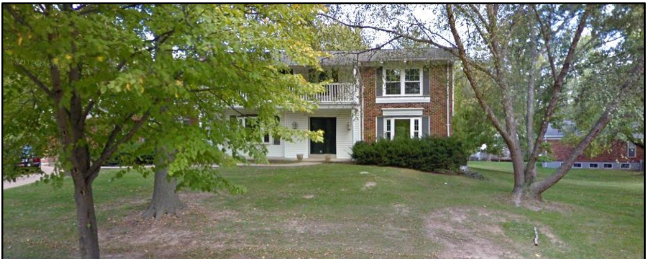
Figure 1: Photo of Subject Site
