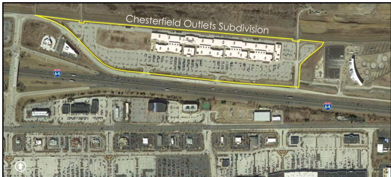
Figure 1: Aerial Site Photo
