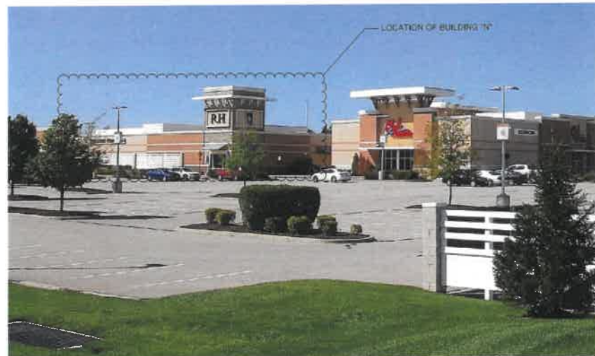
LOOKING NORTH FROM FRONT DRIVE @ NEW BUILDING "N"
