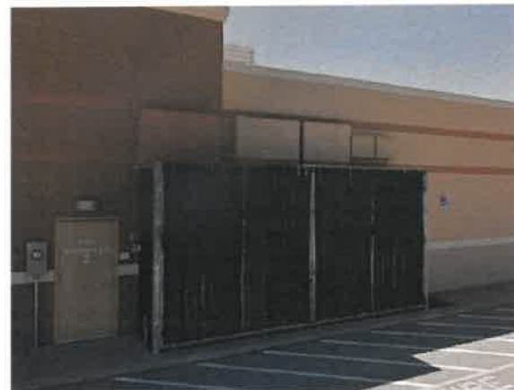
EXISTING SCREENING SYSTEM FOR ELECTRICAL SWITCHGEAR
