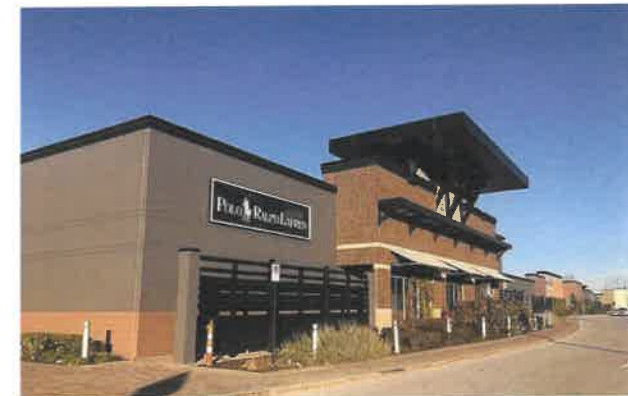
PROGRESS PHOTO - RETAIL BUILDING PAINT UPGRADE (BUILDING "J")
