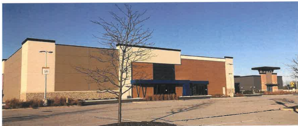
PROGRESS PHOTO - MAIN EVENT (BUILDING "N")
