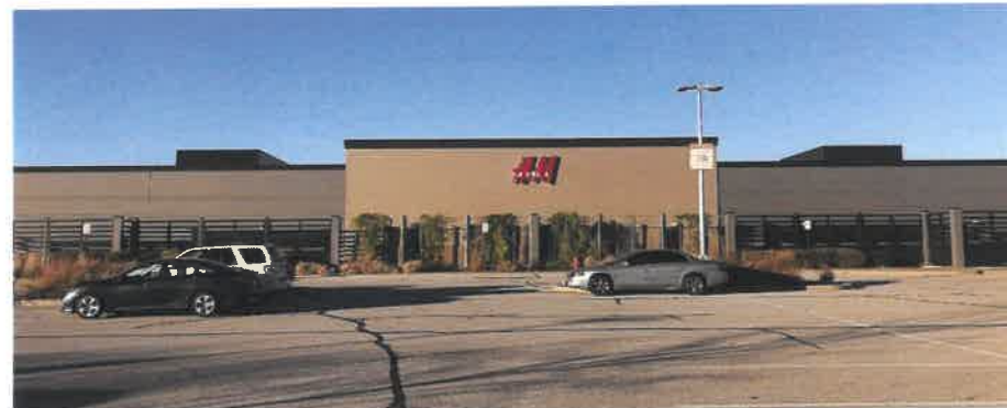
PROGRESS PHOTO - RETAIL BUILDING PAINT UPGRADE (BUILDING "M")
