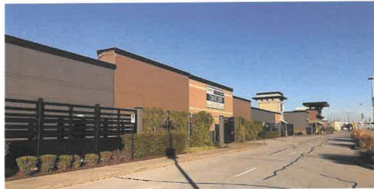
PROGRESS PHOTO - RETAIL BUILDING PAINT UPGRADE (BUILDING "H")
