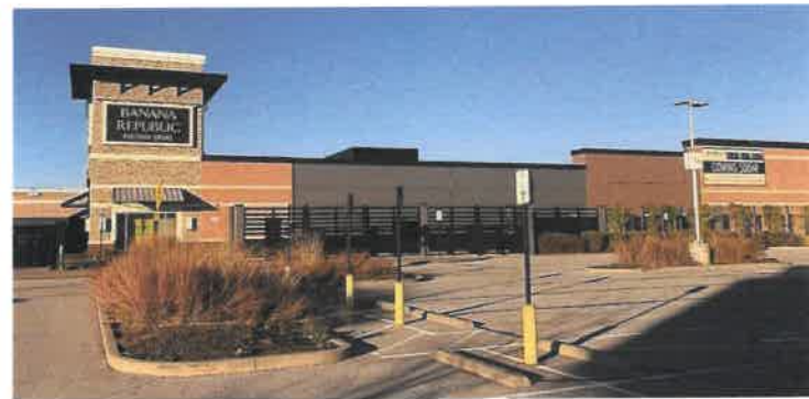
PROGRESS PHOTO - RETAIL BUILDING PAINT UPGRADE (BUILDING "K")
