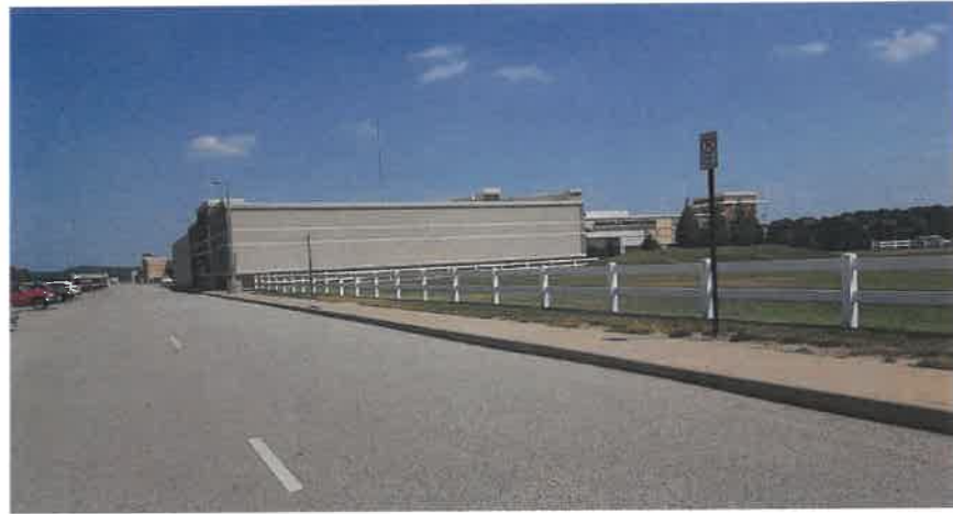
LOOKING SOUTHEAST FROM BACK DRIVE @ NEW BUILDING " C"
