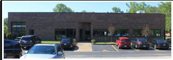
Figure 5: Existing building North side Elevation
