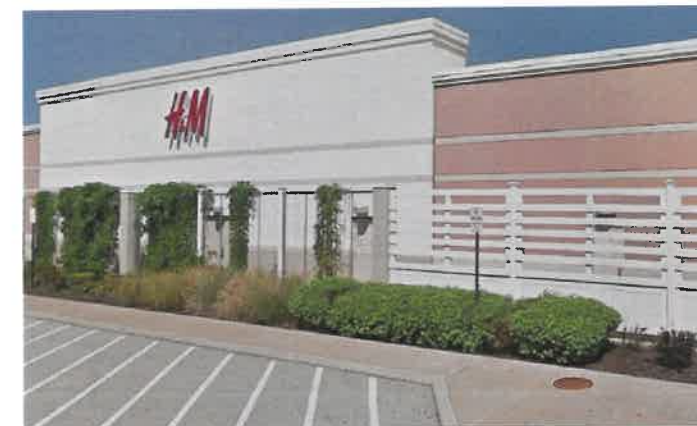
EXISTING SCREENING SYSTEM FOR SOUTH ELEVATION OF DEVELOPMENT AT UTILITY LOCATIONS
