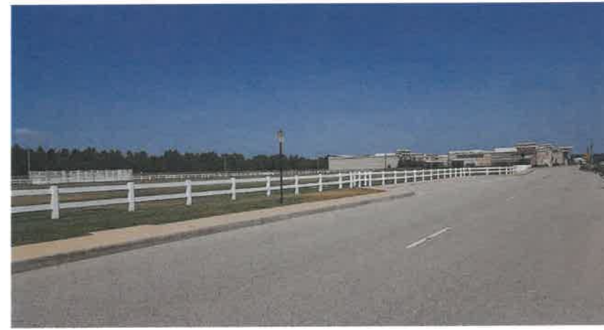
LOOKING NORTHEAST FROM FRONT DRIVE @ NEW BUILDING " C"
