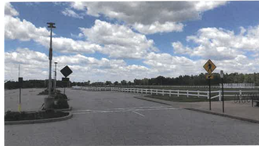
LOOKING NORTHWEST FROM FRONT DRIVE @ NEW BUILDING "C"
