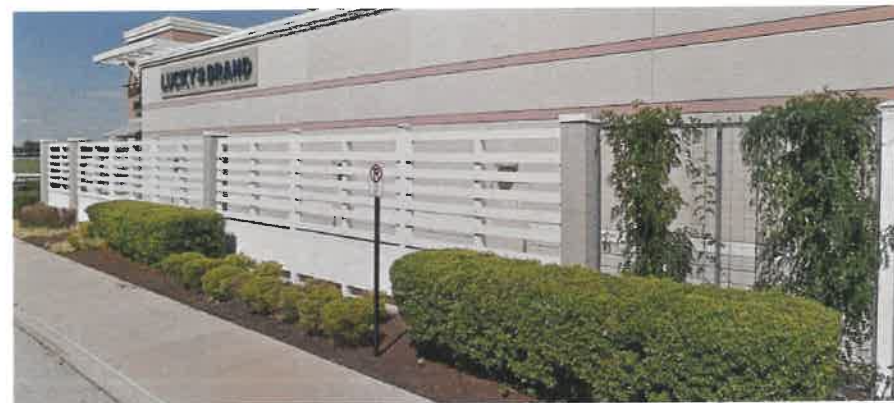
EXISTING SCREENING SYSTEM FOR SOUTH ELEVATION OF DEVELOPMENT AT UTILITY LOCATIONS
