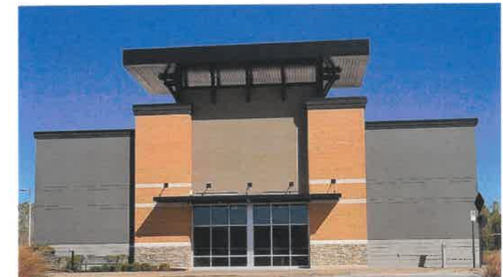
PROGRESS PHOTO - RETAIL BUILDING PAINT UPGRADE (BUILDING "P")
