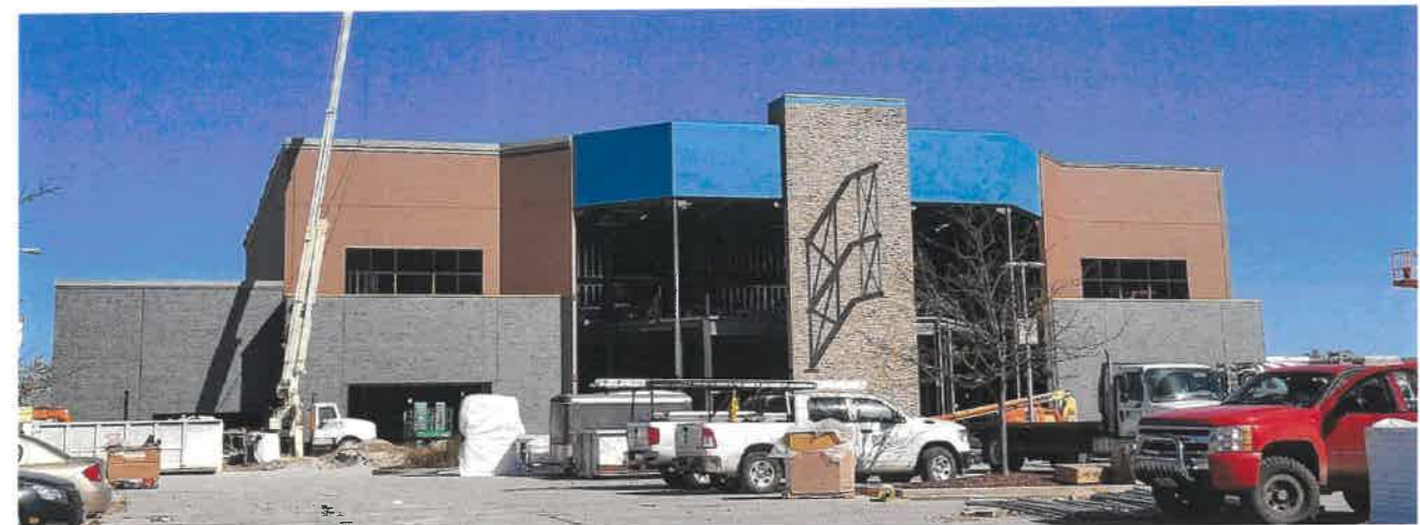
PROGRESS PHOTO - THE FACTORY (BUILDING "C")
