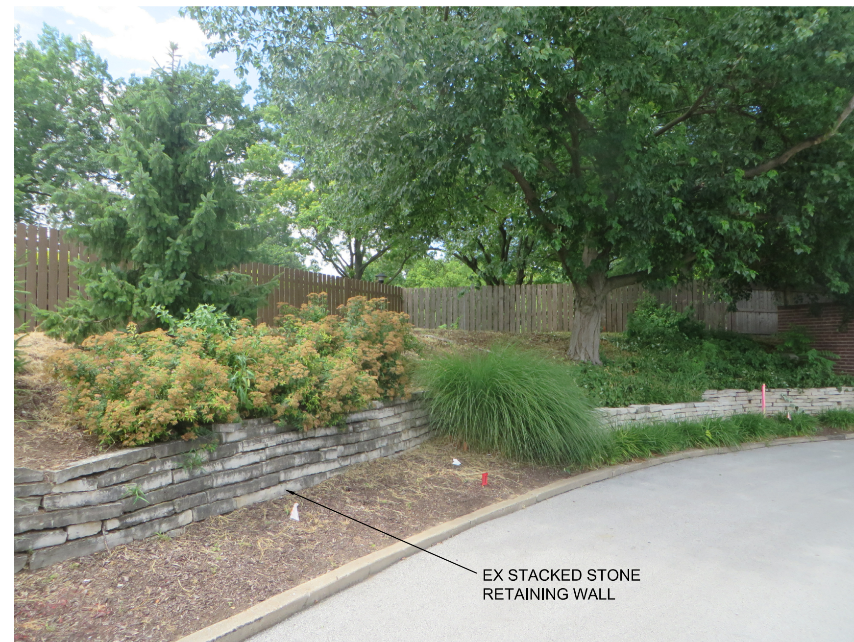
2 EXISTING STACKED STONE RETAINING WALL DETAIL Scale: NOT TO SCALE
