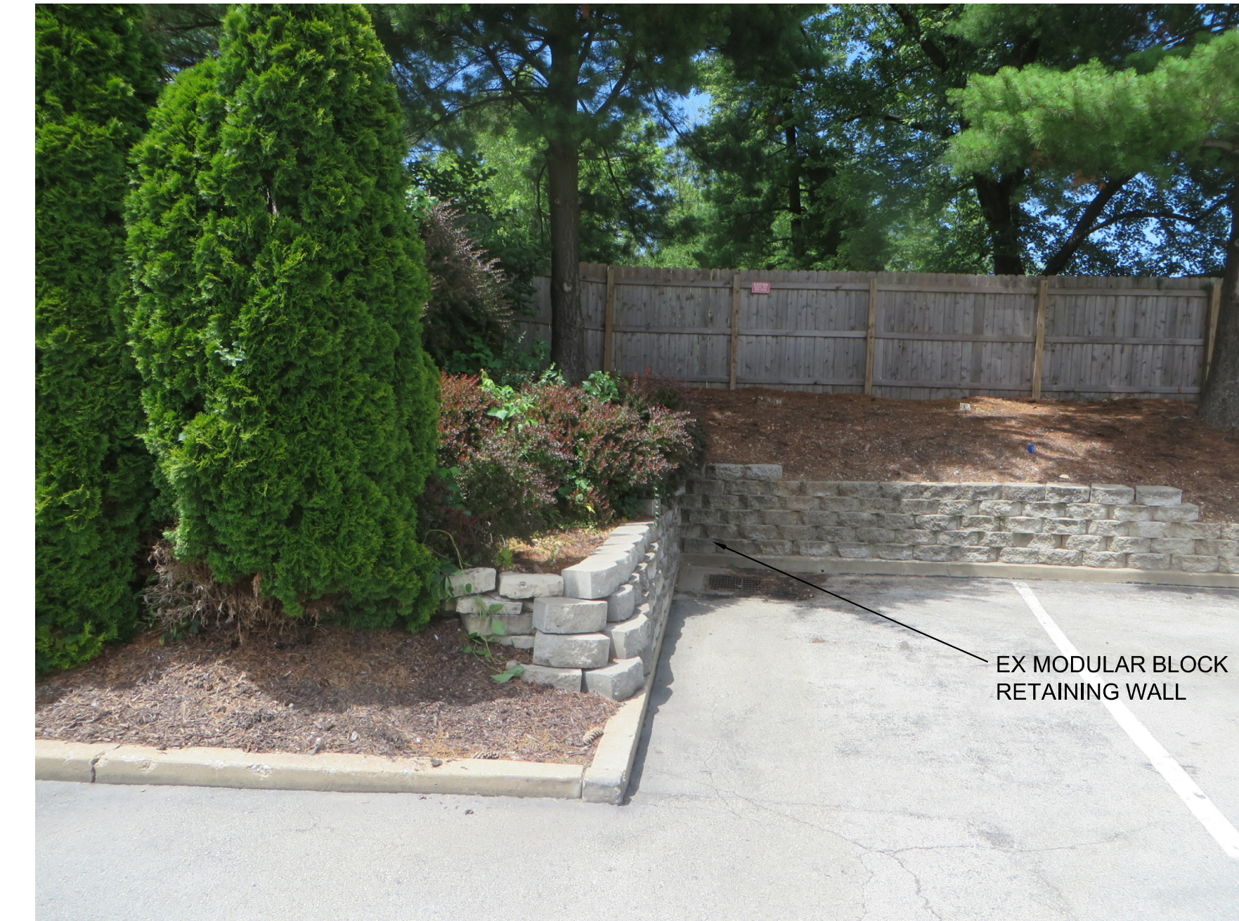
3 EXISTING MODULAR BLOCK RETAINING WALL DETAIL Scale: NOT TO SCALE
