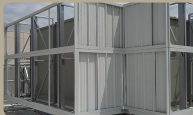
Installation of screen around unit with pipe-chase.
