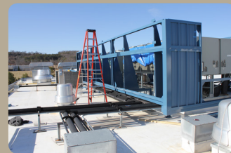
Screen being installed to avoid existing roof piping.
